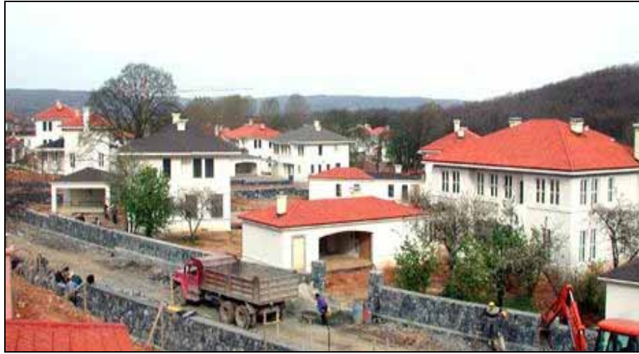
Figure 4.1 A view from a housing estate construction site in Istanbul ( www.arkitera.com )
