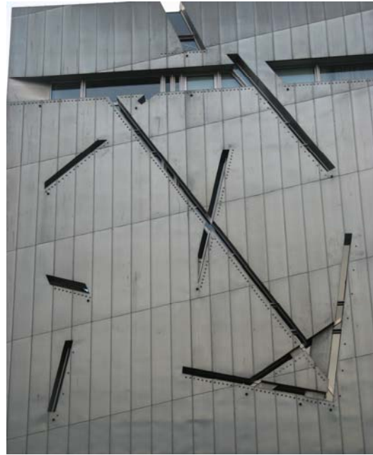
Figure 6.60. Windows on east face of Museum (Photography Feray Maden, December 2006)
