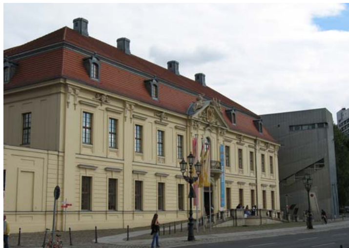
Figure 6.26. Kollegienhaus , the entrance of the Jewish Museum Annex (Photography Feray Maden, August 2007)
