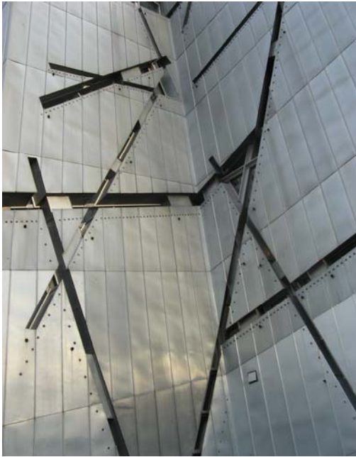
Figure 6.59. Windows on west face of Museum (Photography Feray Maden, December 2006)
