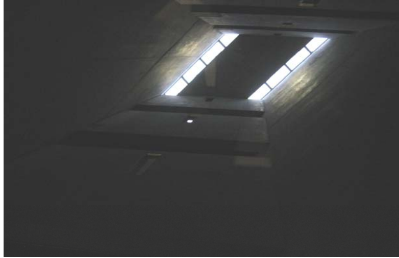
Figure 6.54. Void 3, looking up (Photography Feray Maden, December 2006)
