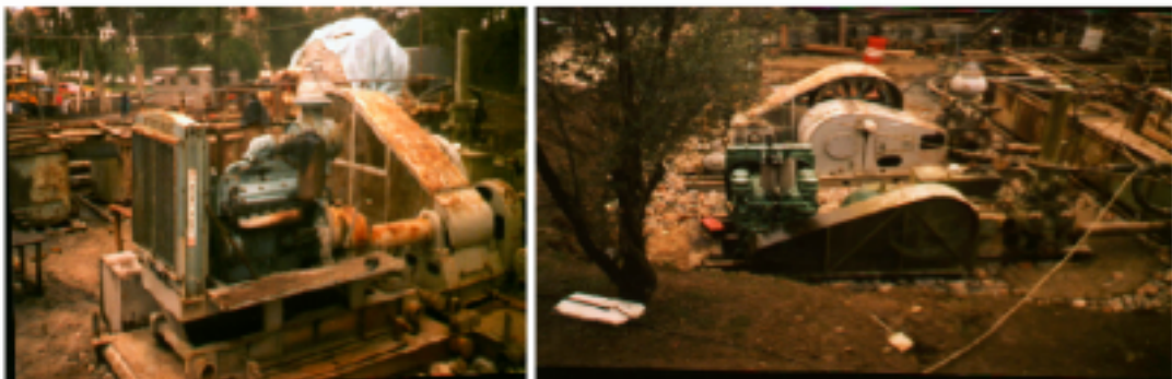
Figure 6.3. Drilling site in BGF
