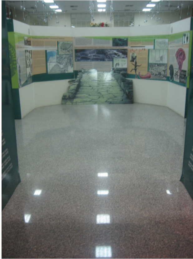
Figure 4.26. Reflected glare from floor under recessed fluorescent lighting
