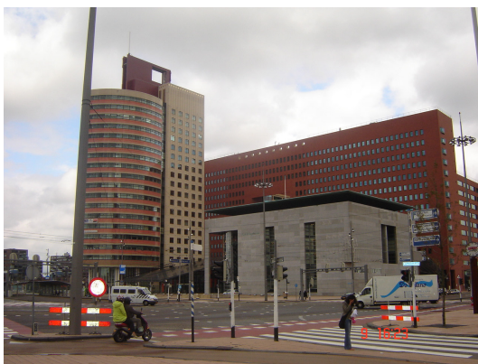
Figure 39. View of Wilhelminaplein (Source: Personal archive)
