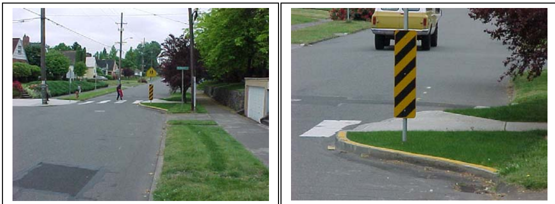
Figure30: Curb extension detail, http://www.transci.portland.or.us
