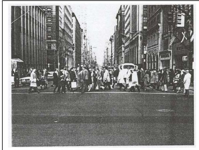
Figure 62: pedestrian space in crosswalks. Unimpeded flow on approaches results in an acceptable space of about 1.80 m 2 Per person on the average in the crosswalk, and about 1.3 m 2 in the middle. (Puskharev, 1978)
