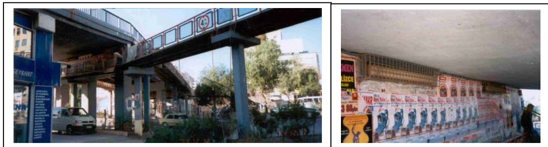
Figure 76: A view to Atilla Altıkat Over Crosswalk and lighting tools
