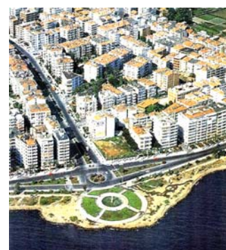
Figure 66. Implementation of coastal road (Metropolitan Municipality Archives)
