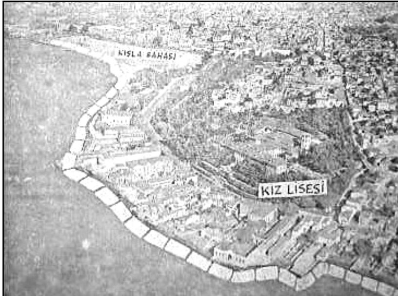
Figure 32. Construction of Konak-İnciraltı Coastal Road (YA, 18.10.1956)
