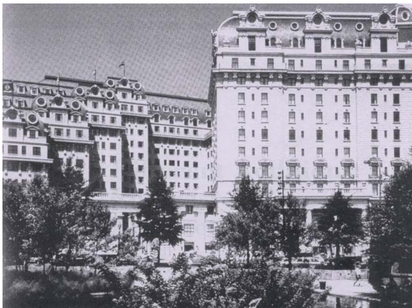
Figure 5.26. Willard Hotel Addition. Mansard roof motifs and fenestration are used to create an appreciative addition (Smeallie and Smith 1990, p.13)
