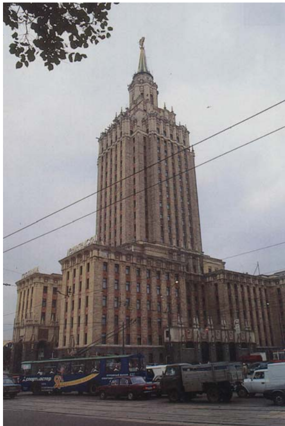
Figure 3.16. One of the skyscrapers of Stalin. Leningradskaya Hotel, by Polyakov, Boretsky, Roçegov (1949-53) The monumentality of scale can be observed (Tanyeli 1999, p.74)
