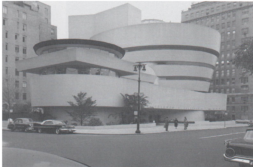
Figure 4.7. Frank Lloyd Wright's Guggenheim Museum, before the addition (Byard 1998, p.142)
