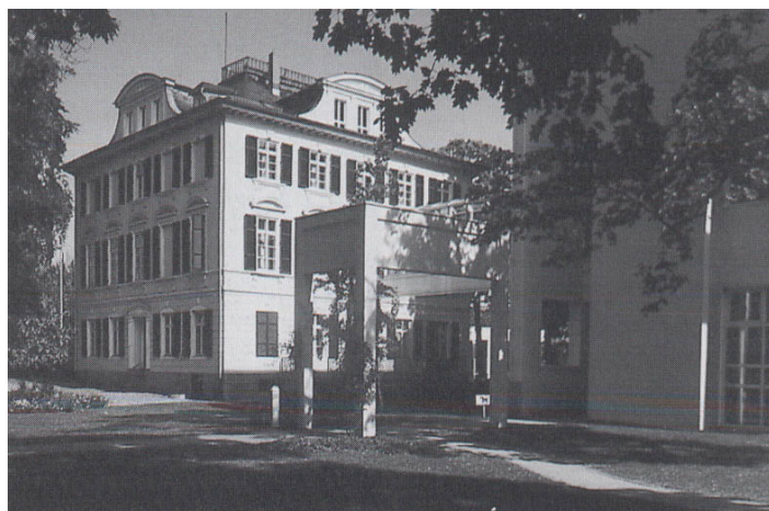
Figure 5.55. Villa Metzler at the entry of the new museum (Byard 1989, p.43)
