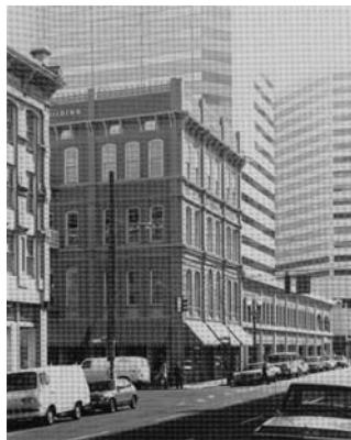
Figure 5.18. Thomas Mann Building – after one and a half story addition and renovation (Dibner A. and Dibner D. 1985, p.27)
