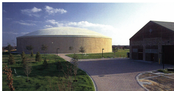
Fig 1.3 Outside view of a chilled water storage tank
