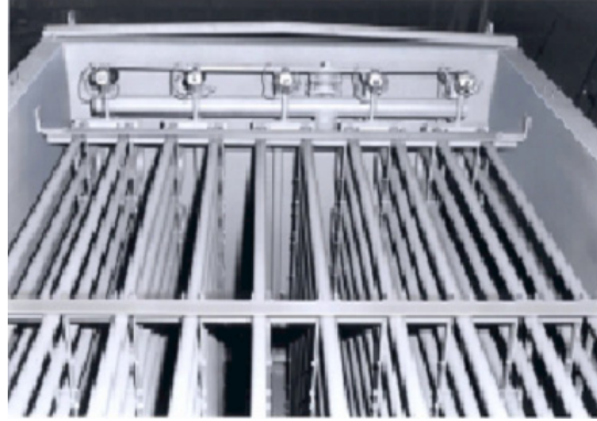
Fig 1.6 External Melt Storage Tank and Internal Piping
