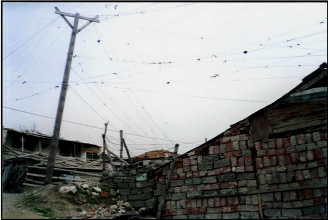
Fig 3.12 : Illegal Tapping of Infrastructure (Electricity), Buca, İzmir
