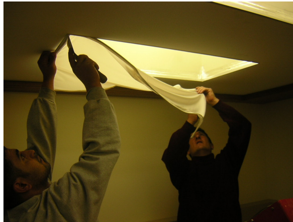
Figure 3.13. Stretching application of PVC.
