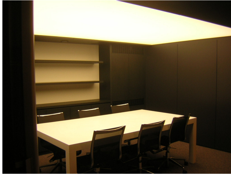
Figure 3.26. Whole ceiling is covered with translucent Barrisol above meeting part of H. Zeki Sungur Office
