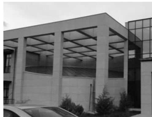
Figure 1. External view of the lecture hall roof.
