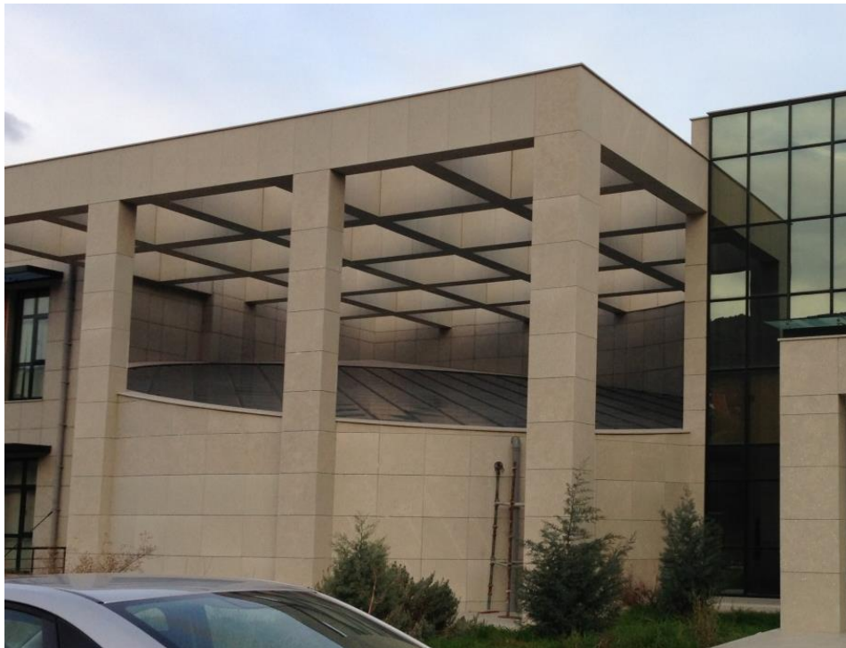
Figure 2. External view of the lecture hall
