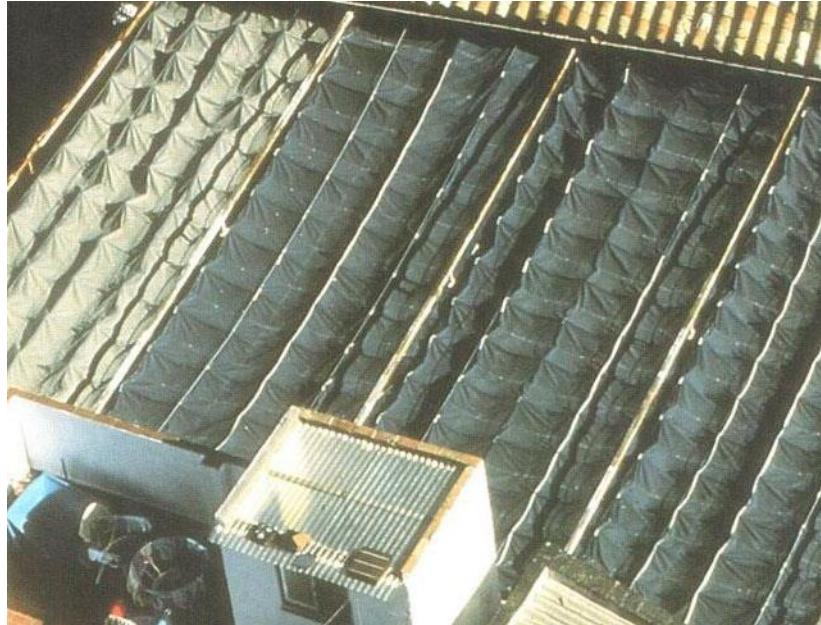
Figure 3.29. Traditional toldos providing shade in the streets of Cordoba, Spain (Source: Otto & Rasch, 1995)
