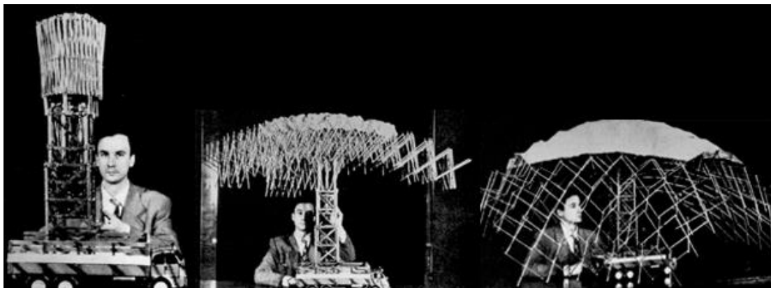
Figure 3.8. Pinero's deployable structure (Source: Robbin, 1996)
