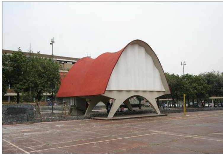
Figure 4.21. The Cosmic Rays Pavilion in Mexico, 1951. Felix Candela's first hyper structure. (Source: Cassinello, 2010)
