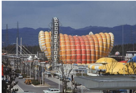
Figure 3.37. Fuji Group Pavilion EXPO '70 Osaka, Japan; is an example for air inflated membrane (Source: Tumblr, 2013)
