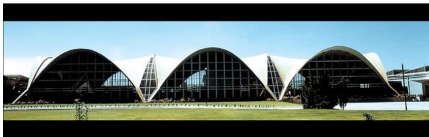
Figure 4.22. Bacardi Rum Factory (1960). (Source: Billington & Garlock, 2010)
