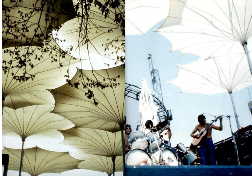
Figure 3.52. Adaptable weather-protection umbrellas for Pink Floyd's USA concert tour in 1977 (Source: Nerdinger, 2005)
