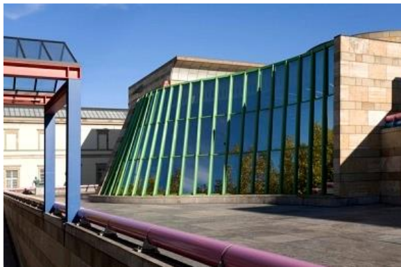
Figure 4.15. The New State Gallery (1977-1983) in Stuttgart by James Stirling (Source: Pottmann, 2007)
