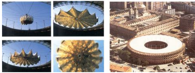
Figure 3.35. Retractable Roof for bullfighting area in Zaragoza, Spain. (Source: Tensinet, 2012)
