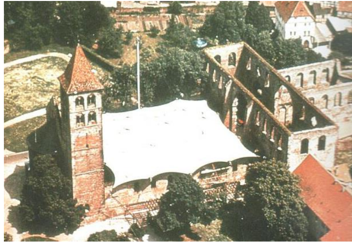
Figure 3.31. Frei Otto's convertible roof design for Bad Hersfeld in 1968 (Source: Otto & Rasch,1995)
