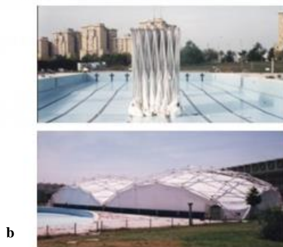
Figure 3.12. a) Model of a Selffolding roof hanging fabric (Source: Escrig et al., 1996) b) The Photo of the deployable roof for San Pablo Swimming Pool (Source: Escrig ,2013)
