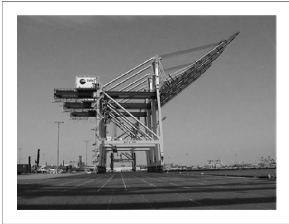
Fig. B.2. A Quay Crane
