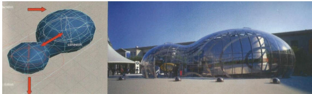
Figure 2. 3. Interaction of two water drops constituting a built form, The Bubble, BMW Exhibition Pavilion, Frankfurt, Germany, Bernhard Franken and ABB Architekten (Source: Kolarevic, 2009)
