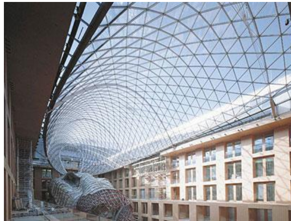
Figure 3. 52. The grid shell, DZ Bank Building, Germany, Frank Gehry & Associates (Source: http://www.gartnersteel.com/content/references/completed_projects/dgb.htm )
