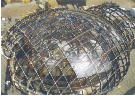
Figure 3. 17. Orthogonal frame layout, The Bubble, Frankfurt, Germany, Bernhard Franken and ABB Architekten (Source: Franken, 2009)
