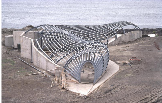
Figure 3. 25. Frame system, H2O Expo Pavilion, Netherlands, Lars Spuybroek (Source: Hadia, 2007)
