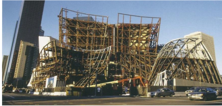
Figure 3. 32. Braced frame system, Disney Concert Hall, LA, California, Frank Gehry (Source: Burry, 2010)
