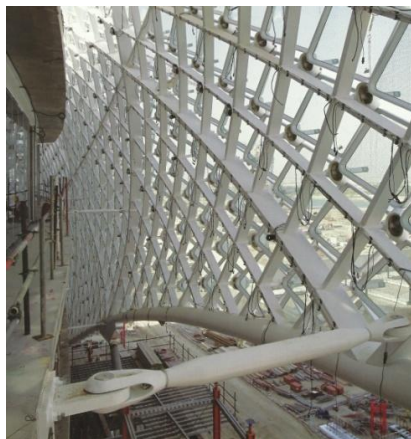
Figure 3. 49. Quadrangular grid of the structure, Yas Hotel, Abu Dhabi, Asymptote Architecture (Source: Burry, 2010)
