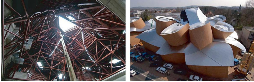
Figure 3. 18. Structural layout and curvilinear outer envelope, MARta Herford Museum, Germany, Frank Gehry (Source: Bagneris, Motro, Maurin, Pauli, 2008)
