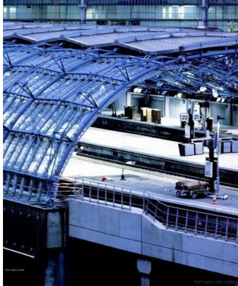
Figure 4. 15. Primary and secondary structural elements (Source: Riley, 1995)
