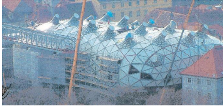
Figure 4. 8. Various sized triangles over the surface during construction (Source: Project Building Info, 2013)
