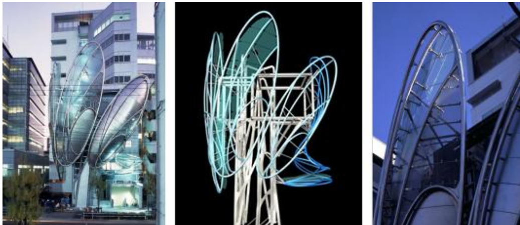
Figure 2. 5. The wing above ground (Source: http://www.makoto-architect.com/subway/subway_2e.html )
