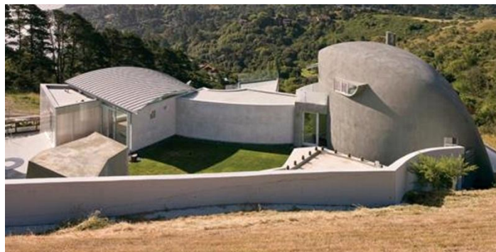
Figure 3. 60. Solid shell structure, California Bay House, San Francisco, Leonard and Walker & Moody Architects (Source: Composites Technology, 2010)
