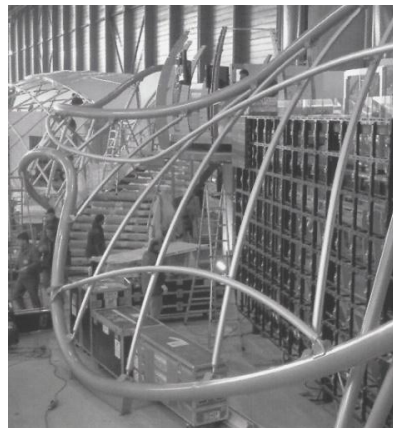
Figure 3. 56. Grid system in detail, Brandscape BMW Pavilion, Geneva, Switzerland, Bernhard Franken and ABB Architekten (Source: Franken, 2009)
