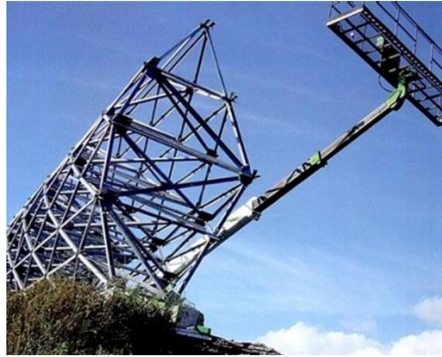
Figure 3. 40. Space frame of the Acoustic Barrier, Utrech, Holland, Kas Oosterhuis (Source: Oosterhuis, 2008)
