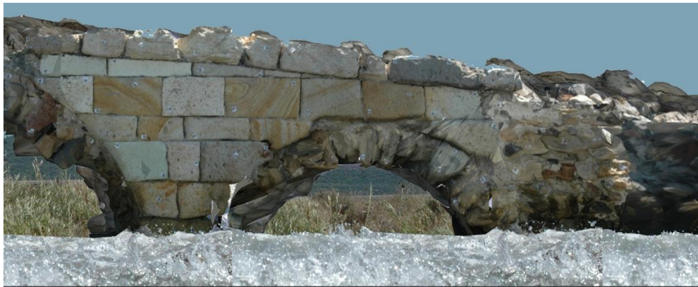
Downstream (Northern Facade)
