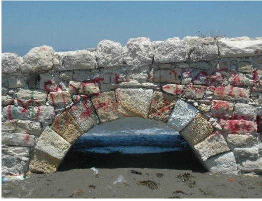
Flat spandrel walls; Hypokremnos Projected spandrel walls; Babaeski Viaduct Viaduct (Seljukid Period)
