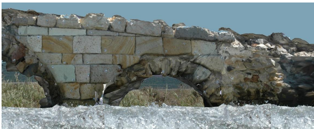
Downstream (Northeastern) Facade
