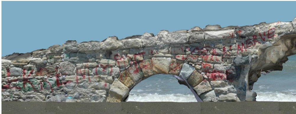
Upstream (Southwestern) Façade
