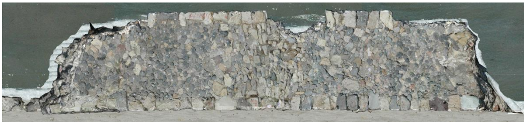
Figure 4.10. Floor covering of Hypokremnos Viaduct
