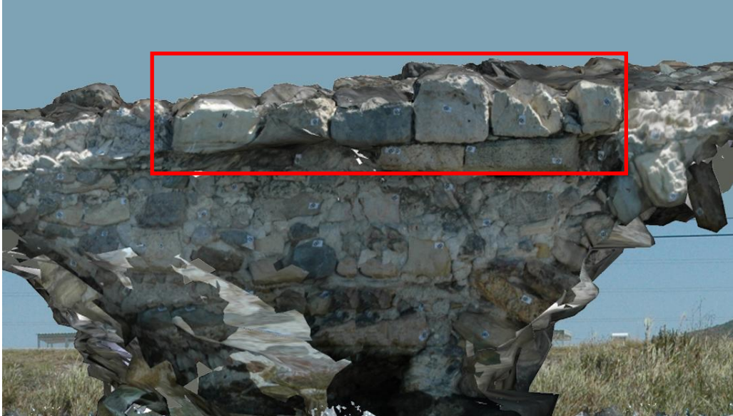
Figure 3.16. Parapet walls
