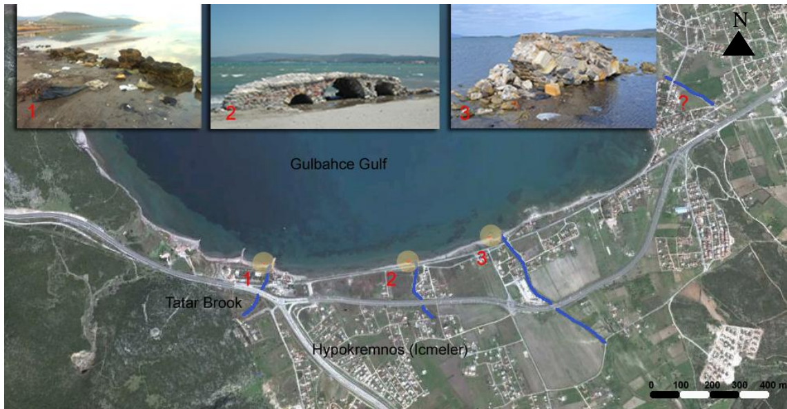
Figure 3.9. Location of the Hypokremnos Viaducts
