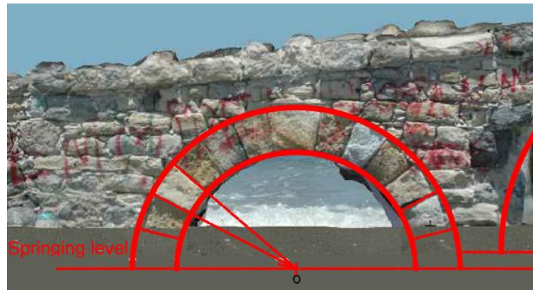
Figure 3.14. Semicircular arch and keystone in the smallest arch
