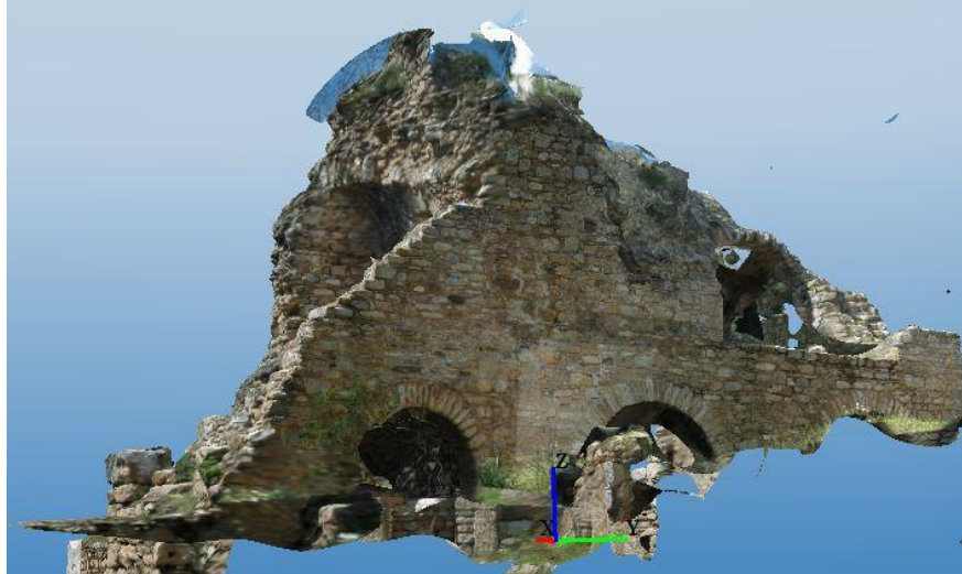
Figure 3.37. Model of rubble stone facing
