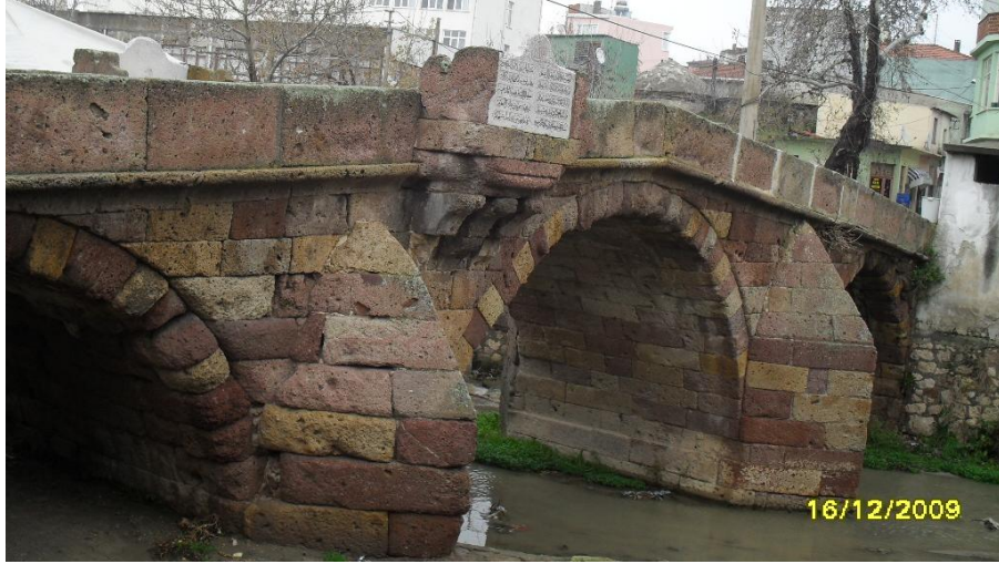
Figure 4.5. Different coloured and sized cut stone blocks in a Seljukid Viaduct; Bayramiç Viaduct (Source: Çanakkale İli Private Website 2009)
