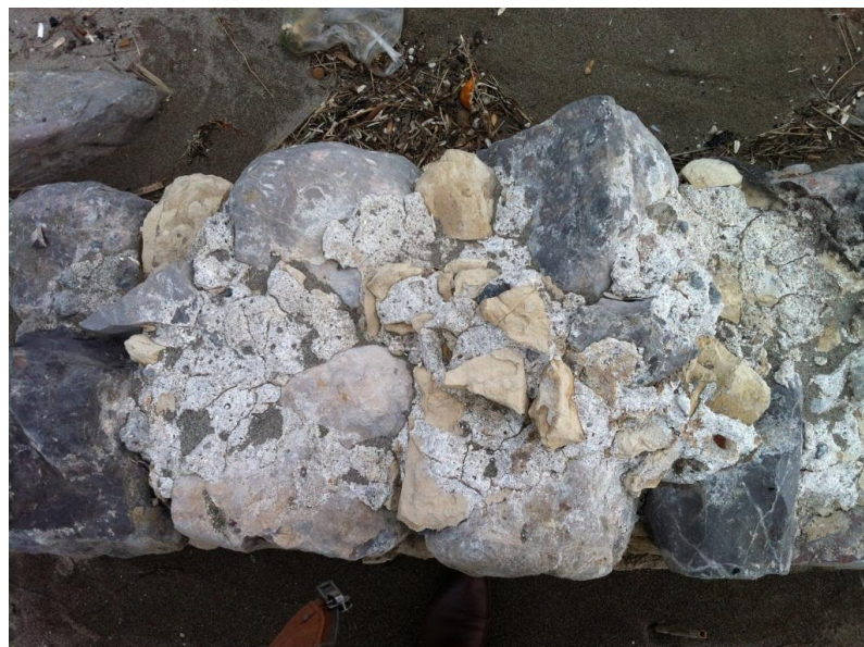
Figure 3.12. Double layered facing stones of the viaduct
