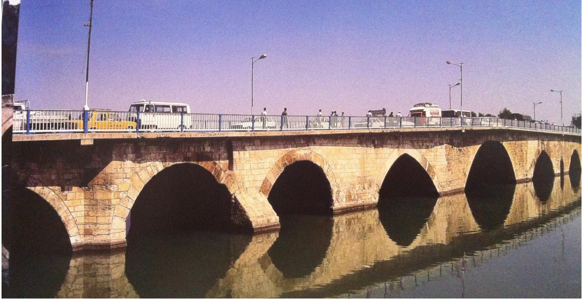
Figure 4.3. A rectangular formed Roman Viaduct; Taş Viaduct, Seyhan, Adana (Source: Tanyeli 2000)
