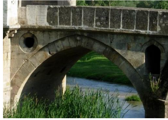
Flat spandrel walls; Hypokremnos Projected spandrel walls; Babaeski Viaduct Viaduct (Seljukid Period)
