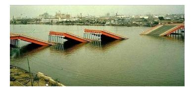
Figure 2.10. Lateral Spreading Problem After the 1964 Niigata Earthquake (Source: www.ce.washington.edu)
