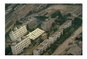
Figure 2.11. Bearing Capacity Problem After 1964 Niigata Earthquake (Source: www.ce.washington.edu)
