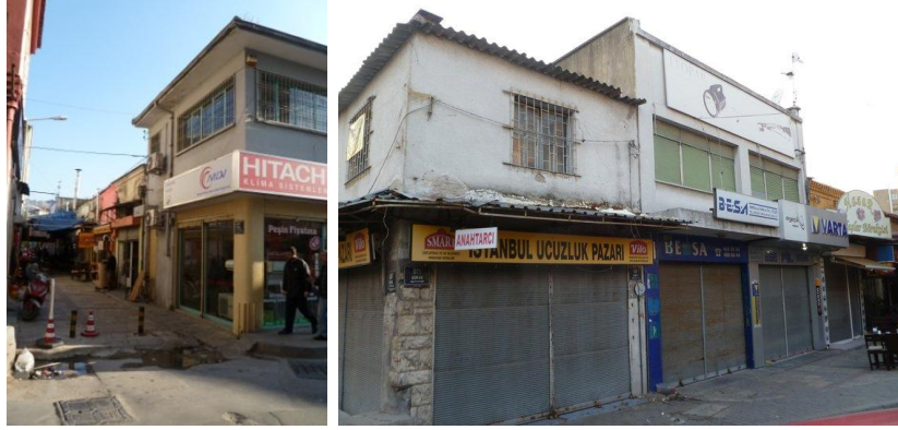
Figure 28. Views of the northeastern facade on 897 Street (Source: Palaoğlu 2011)
