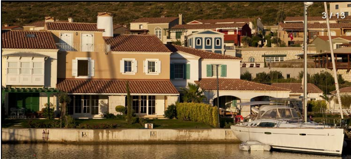
Figure 30. A View from the Port Alaçatı Project (Source: http://portalacati.com.tr/galeri/galeri.aspx )
