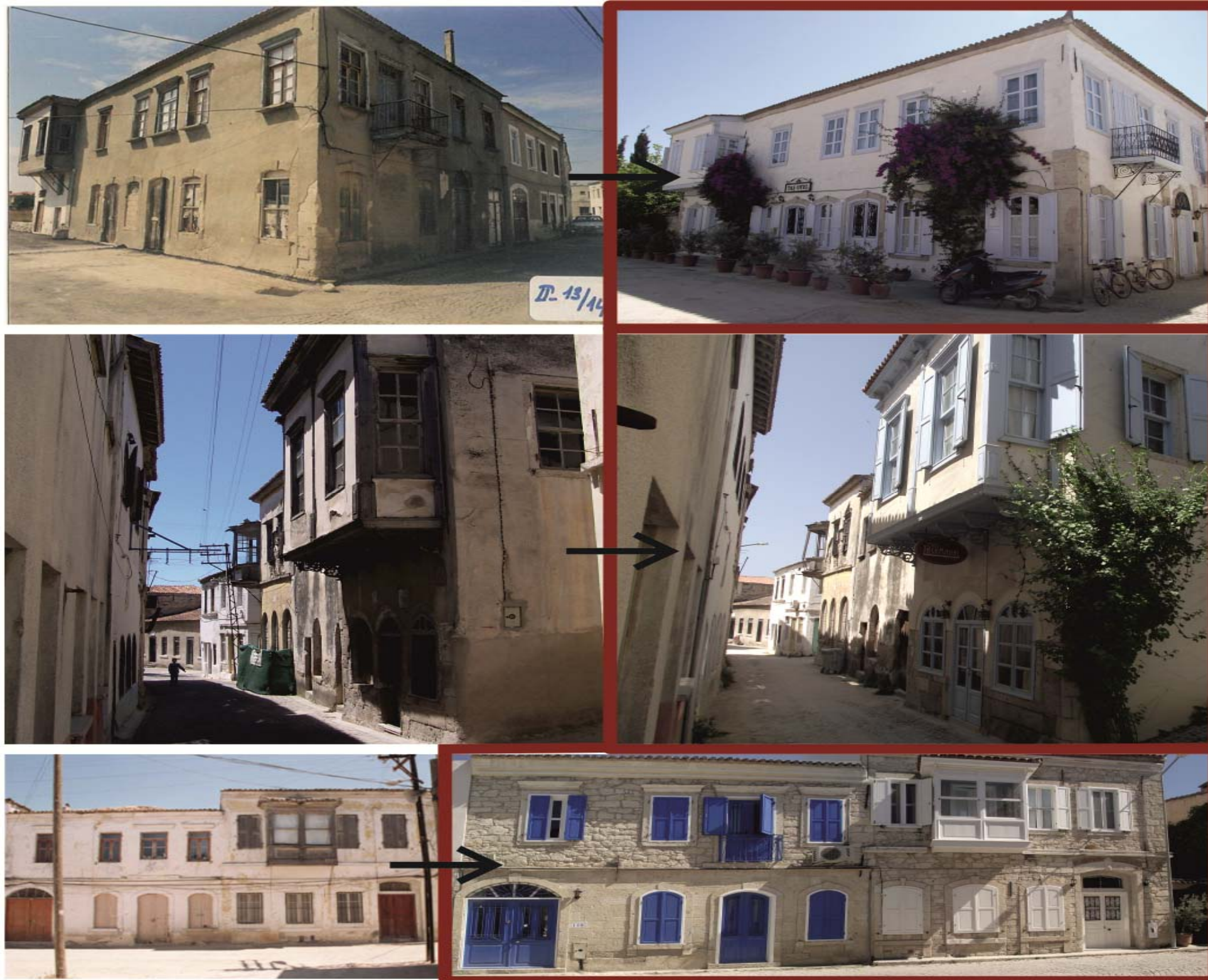
Figure 38. Before and After Cases of Some of the Traditional Buildings (Pictures in the left hand side: the Archive of the Alaçatı Municipality; Picture from the right hand side: the Author's Archive, July-August 2011)
