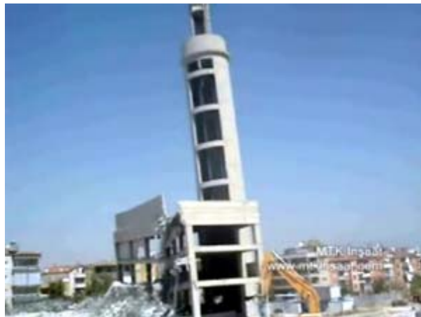
Figure 47. The Facility While Being Demolished (Source: Wowturkey/6, 2010)
