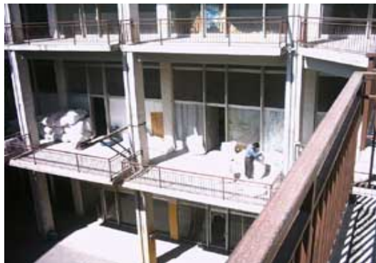
Figure 13. A view from the Vacant Shop
