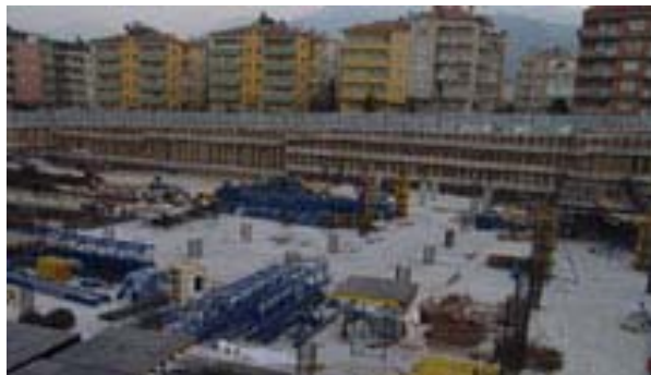
Figure 48. Ground floor of the construction
