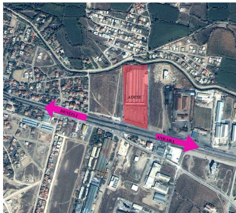
Figure 16. Satellite View of Adese Shopping Center (Source: Denizli Municipality, 2007)
