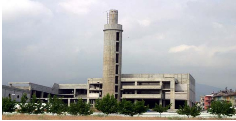
Figure 17. View from the Construction
