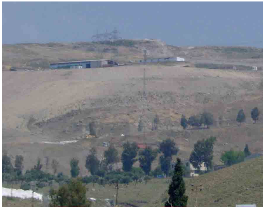
Figure 3.15 Harmandalı municipal solid waste separation facility
