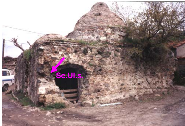
Figure 3.8 View from the southwest elevation of the Ulamiş Bath in Seferihisar, showing where stone masonry mortar samples (Se.Ul.s.) were collected.
