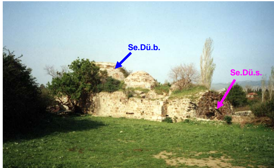
Figure 3.4 View from the southeast and southwest elevations of the Düzce Bath in Seferihisar, showing where stone masonry mortar samples (Se.Dü.s.) and brick masonry mortar samples (Se.Dü.b.) were collected.
