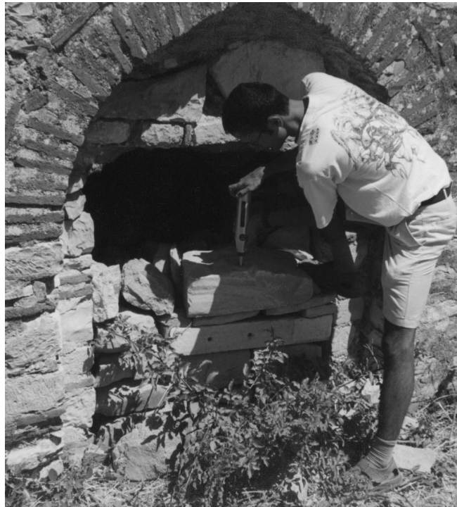
Figure 4.21 Schmidt Hardness tests on stone S1, insitu.
