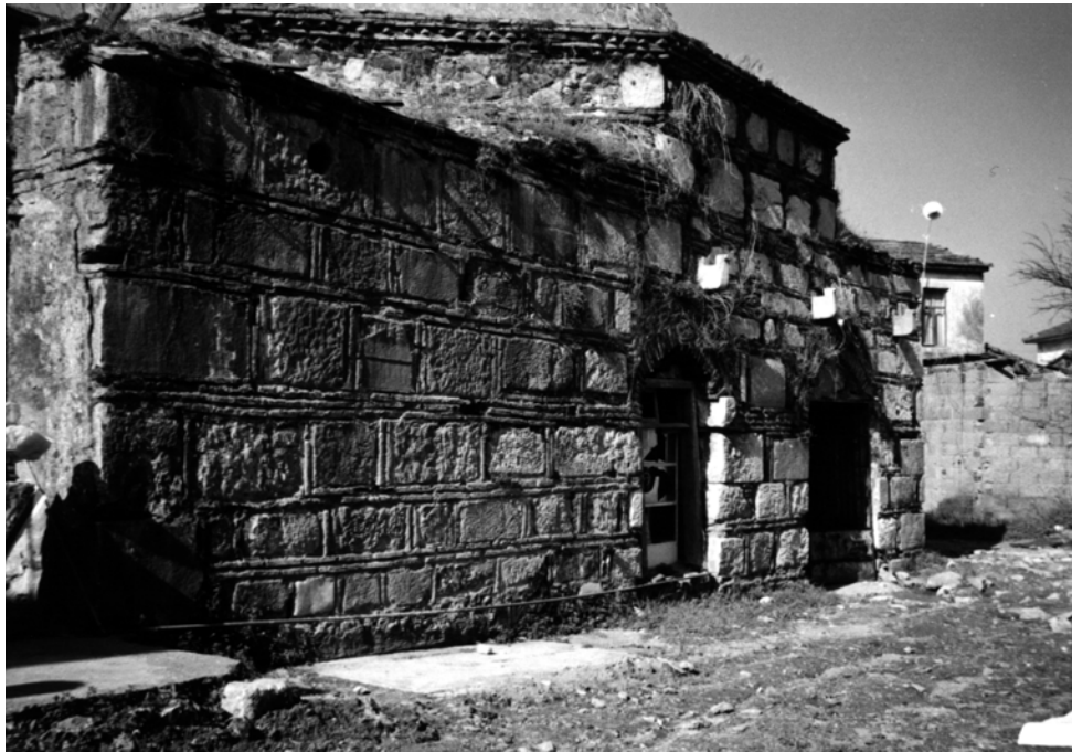
Figure 3.22. Seferihisar Büyük Hamam, Reused Cut Stone / Brick Alternating Bond of the Entrance Facade.
