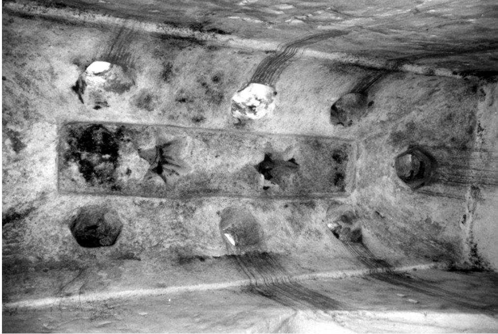
Figure 3.25. Seferihisar Büyük Hamam, The Panelled Vault in the Side Sections of the Main Sıcaklık Space
