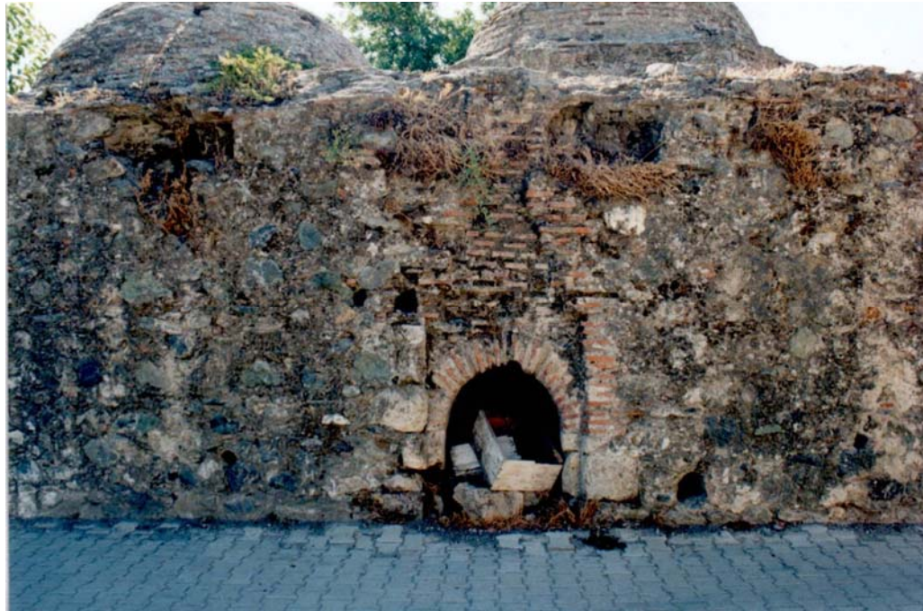
Figure 3.3. Ulamiş Hamamı, The Entrance of the Hamam from the West
