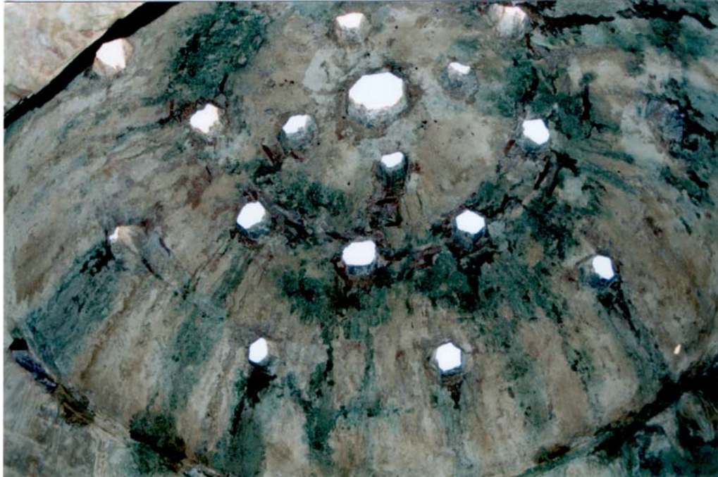
Figure 3.19. Düzce Hamamı, The Dome and Use of Oculi on the Dome of Main Sıcaklık Space
