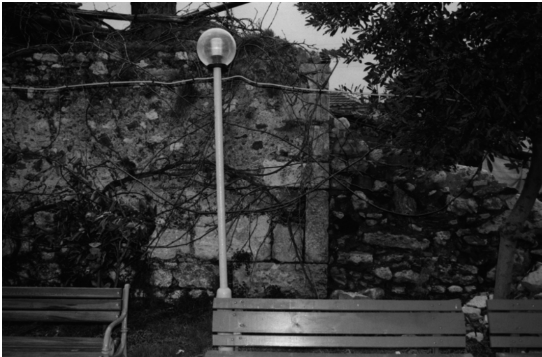
Figure 3.36. Sığacık Kaleiçi Hamamı, The Northeast Facade, The Use of Reused Cut Stone in Vertical Line
