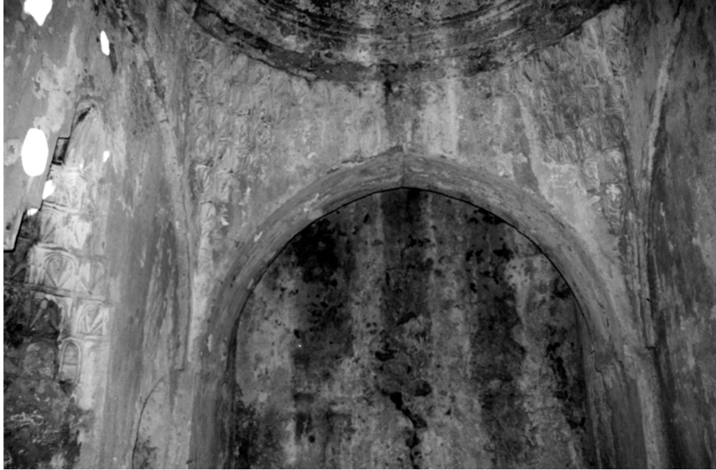
Figure 3.54. Urla Kamanlı Hamamı, The Muqarnas Decorated Pendentives in the Main Sıcaklık Space
