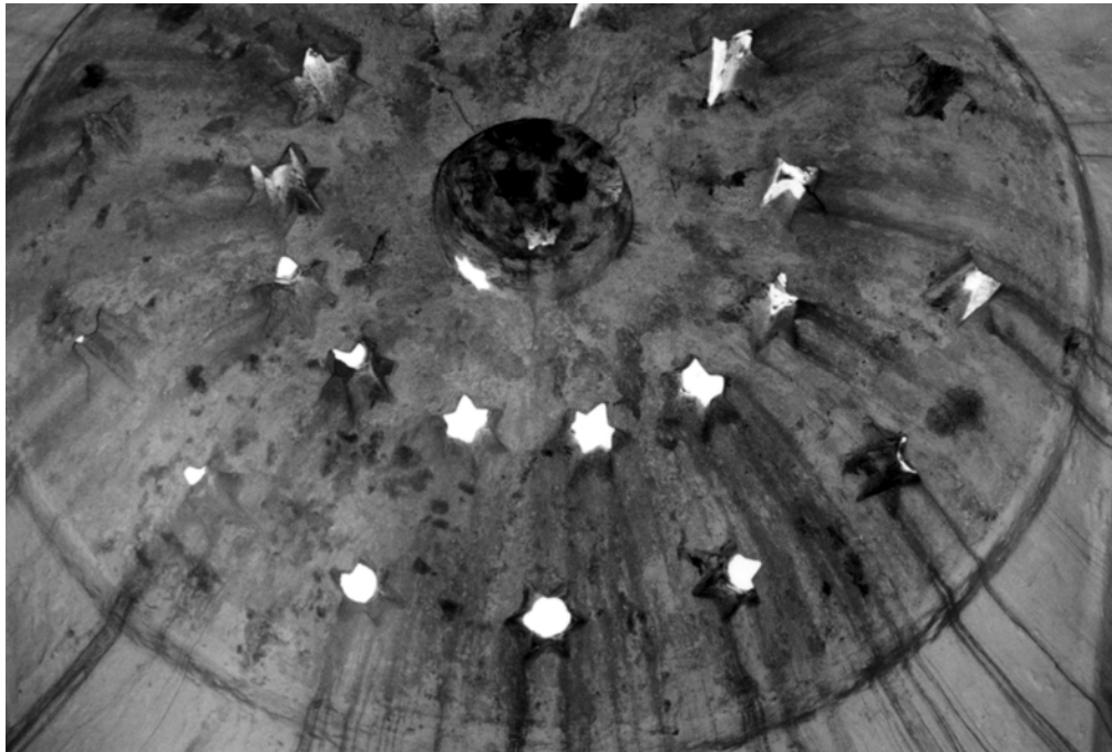
Figure 3.26. Seferihisar Büyük Hamam, The Use of Oculi and Hemispherical Cupola on the Dome of Main Sıcaklık Space
