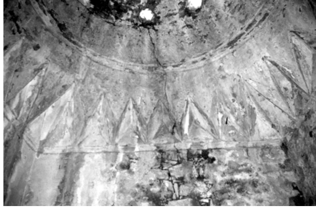
Figure 4.17. Urla Kamanlı Hamamı, Belt of Turkish Triangles in the Northwest Halvet
