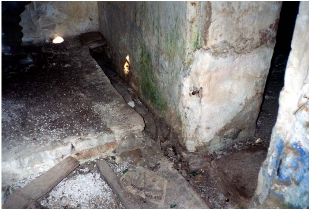
Figure 3.69. Urla Özbek Hamamı, The Waste Water Channels in the Ilıklık Space
