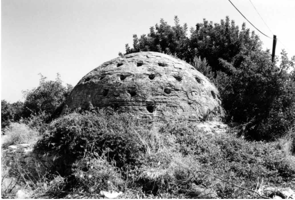
Figure 3.62. Urla Rüstem Paşa Hamamı, The Dome of the Existing Space
