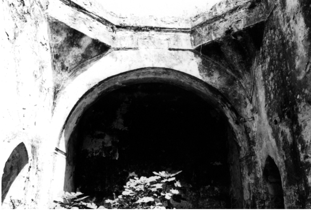
Figure 3.44. Urla Çifte Hamam, Pendentives in the Main Sıcaklık Space of Men's Section
