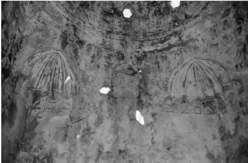
Figure 3.53. Urla Kamanlı Hamamı, The Lobed Squinches in the East Halvet
