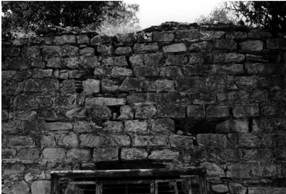
Figure 3.51. Urla Kamanlı Hamamı, The West Exterior Wall
