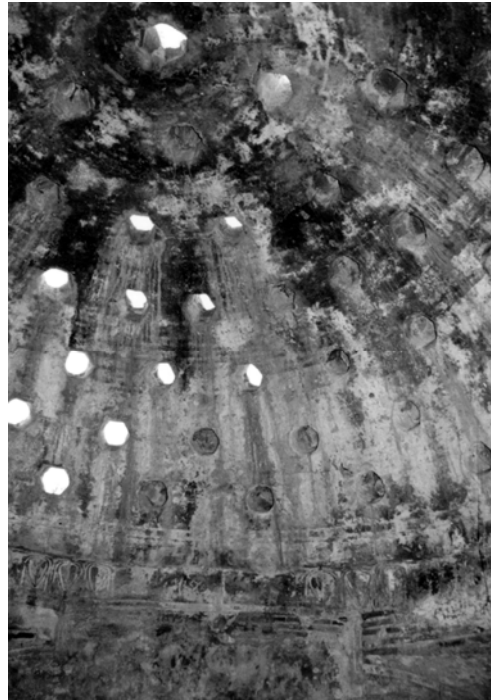
Figure 3.63. Urla Rüstem Paşa Hamamı, The Oculi on the Dome of the Existing Space
