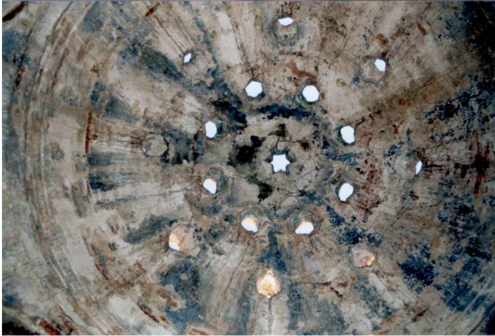
Figure 3.8. Ulamiş Hamamı, The Use of Oculi on the Dome of the West Halvet
