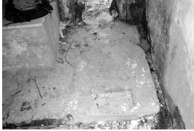
Figure 4.21. Seferihisar Küçük Hamam, Waste Water Channel in the Ilıklık Space
