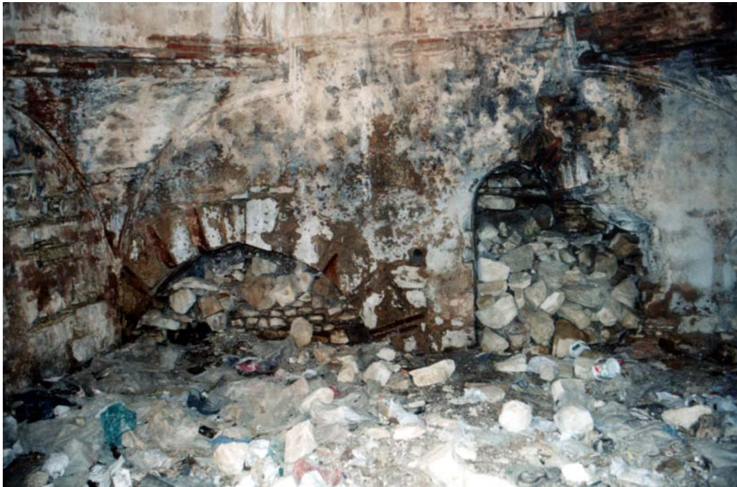
Figure 3.61. Urla Rüstem Paşa Hamamı, Arches and Pendentives in the Existing Space
