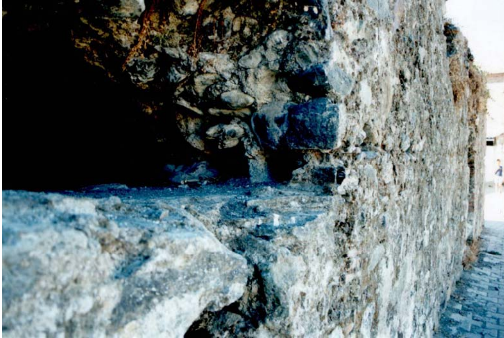
Figure 3.6. Ulamiş Hamamı, The Timber Beams in the Walls
