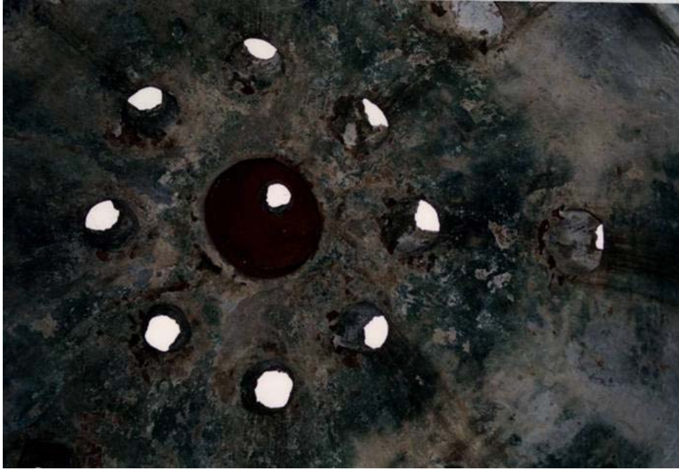
Figure 3.32. Seferihisar Küçük Hamam, The Oculi and Cupola on the Dome of the West Halvet
