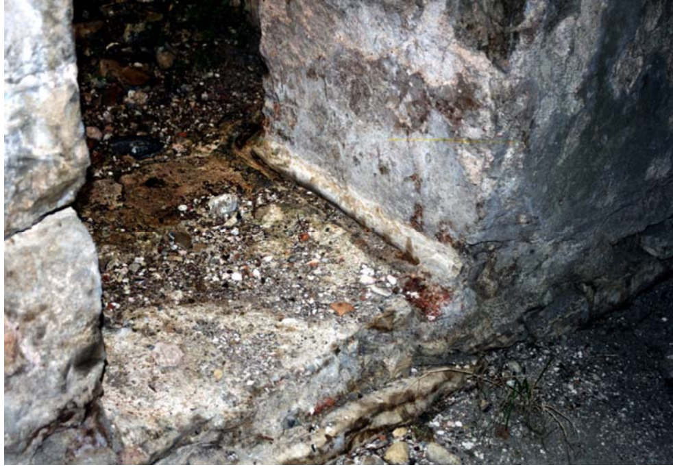
Figure 3.58. Ural Kamanlı Hamamı, The Traces of Waste Water Channel on the West Edge of the Door Opening between the Ilıklık and the Main Sıcaklık Space
