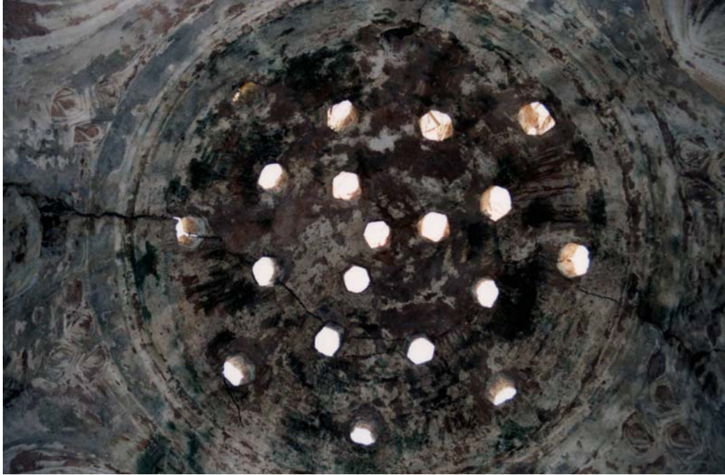
Figure 3.56. Urla Kamanlı Hamamı, Oculi on the Dome of the East Halvet
