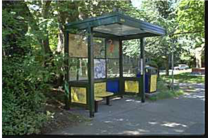
Figure 3. 16. ‘Green’ Bus Shelter
