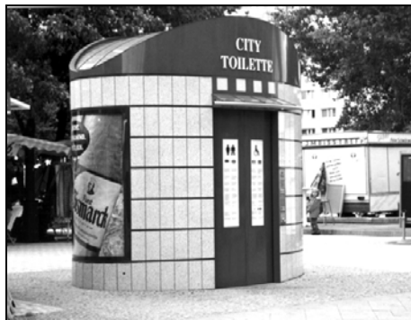
Fig. 4.4. Public Sanitary Unit
