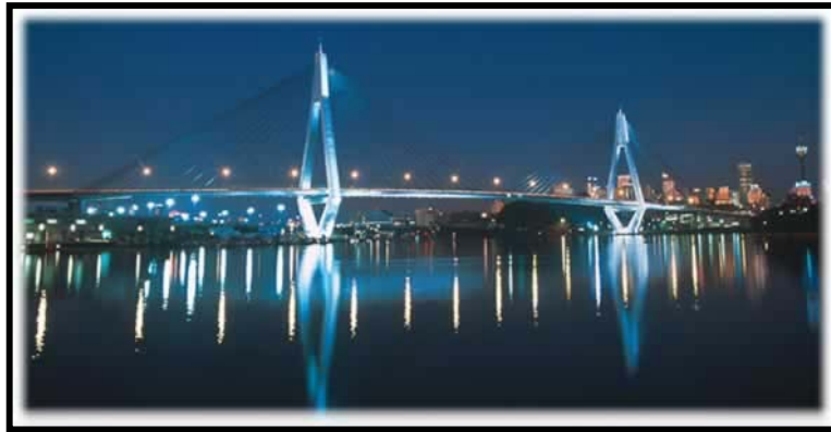
Figure 3.26. Illumination of Anzac Bridge (Source: Philips, Issue No:8 2001)
