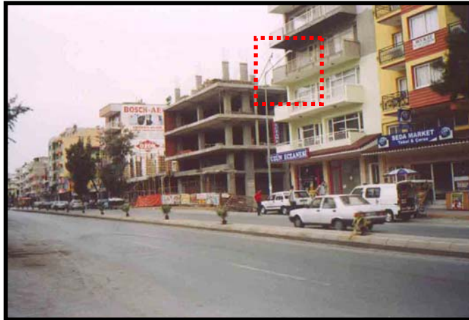
Figure 4.2 The existing installation causes the light trespass in Narlıdere.
