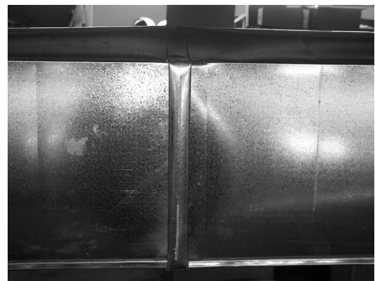
Figure B12. Drive Slip J. under Pressure
