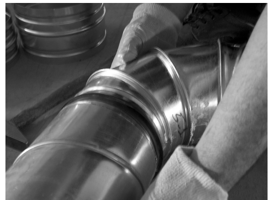
Figure B4. Assembly of An Elbow
