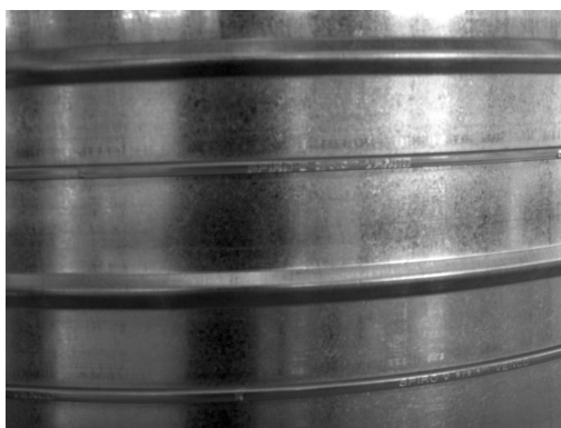
Figure B5. Corrugation in a Circular Duct
