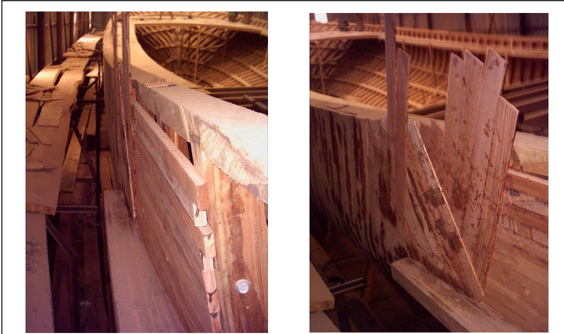
Figure 4.60. Laminating views of hull of a Gulet. (Gölpınar 2004)
