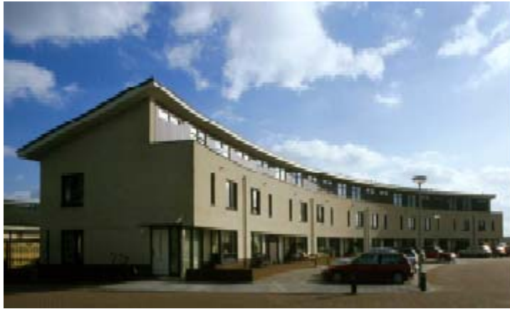
Figure 1.5: The one-family terrace houses in Harderwijk.
