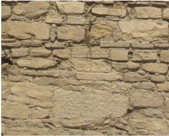
Figure 4.31. Progress of the efflorescences and discharge of mortar between the years 2004-2005
