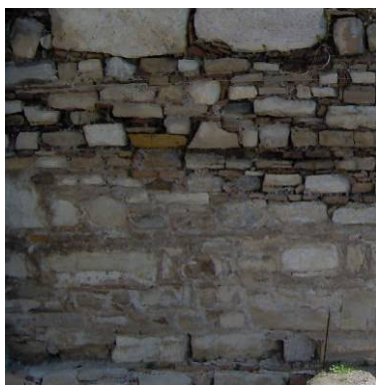
Figure 3.17. Soiling
