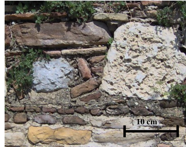
Figure 4.30. Progress of the black crust, biological colonization and discharge of mortar between the years 2002-2005
