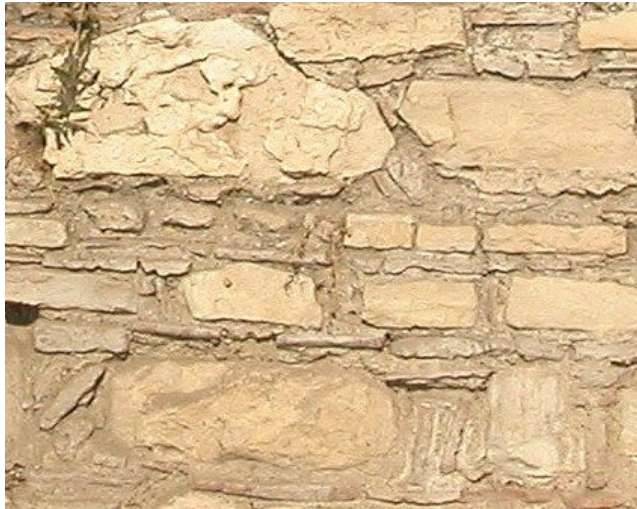
Figure 4.37. Progress of the black crust and discharge of mortar between the years 2003-2005
