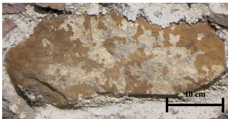
Figure 3.18. Colored crust tracing the surface
