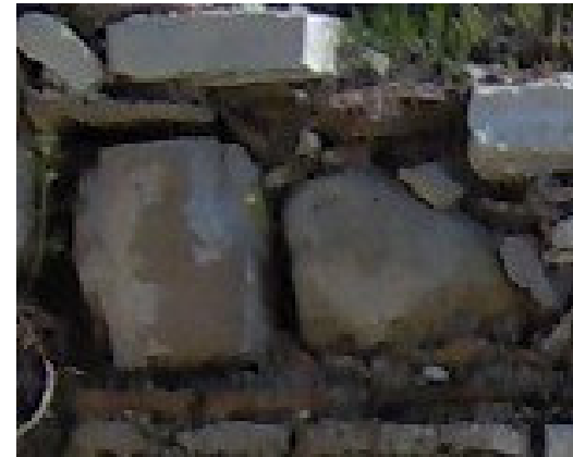
Figure 4.33. Progress of the black crust and biological colonization between the years 2002-2005
