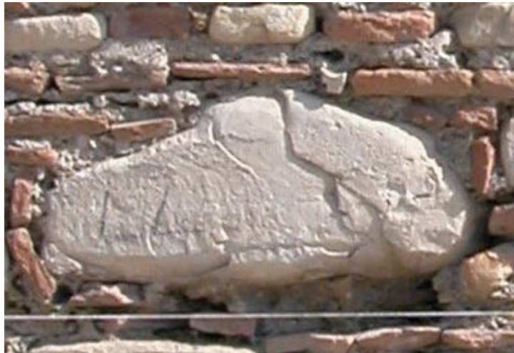
Figure 4.31. Progress of the efflorescences and discharge of mortar between the years 2004-2005
