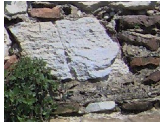
Figure 4.33. Progress of the black crust and biological colonization between the years 2002-2005
