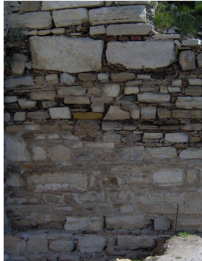
Figure 4.28. Progress of discharge of mortar, efflorescences and rounding between years 2003-2005 in the bastion three
