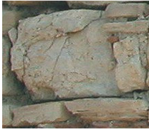
Figure 4.35. Progress of the splintering between the years 2003-2005
