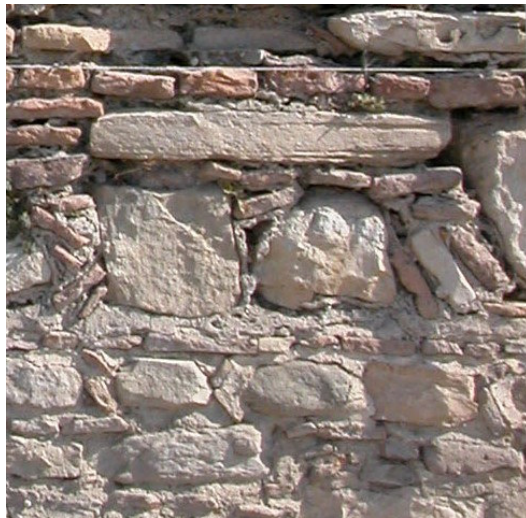
Figure 4.36 Progress of the black crust, biological colonization and discharge of mortar between the years 2002-2005
