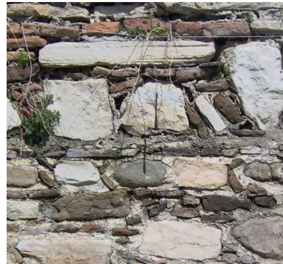
Figure 4.36 Progress of the black crust, biological colonization and discharge of mortar between the years 2002-2005
