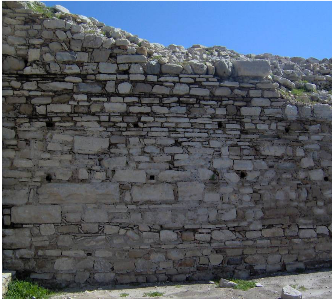
Figure 4.27. Progress of efflorescences and discharge of mortar between the years 2003-2005 in the city wall between 4. and 5. bastions
