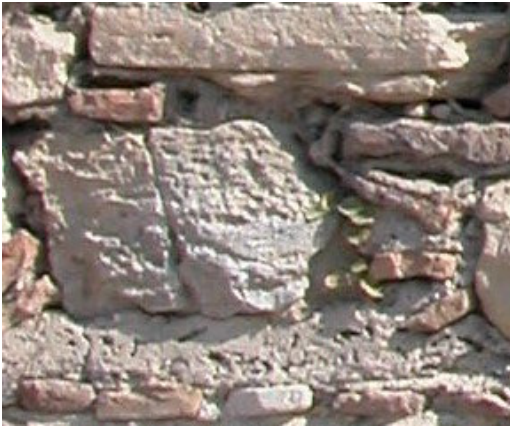
Figure 4.33. Progress of the black crust and biological colonization between the years 2002-2005
