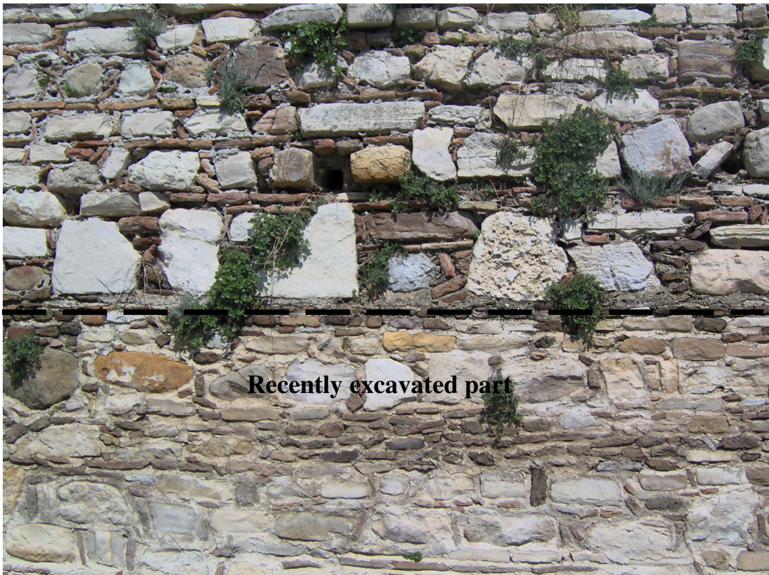
Figure 4.20. Coloration, biological colonization and black crust.
