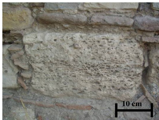
Figure 3.7. Alveolar weathering
