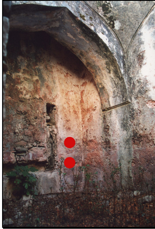
Figure 3.13. Kamanlı Bath, ılıklik space, showing where the samples were collected
