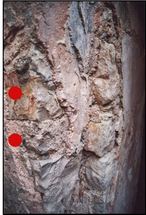
Figure 3.11. Hersekzade Bath, sıcaklık space, showing where the samples were collected
