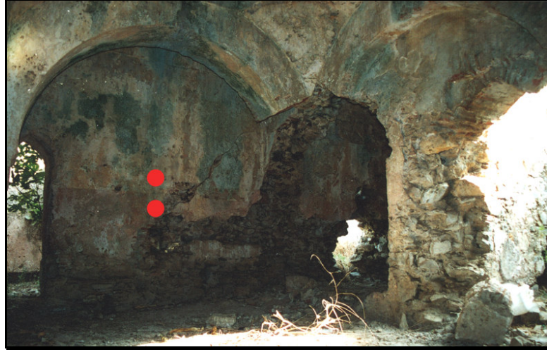
Figure 3.17. Düzce Bath, ılıklik space, showing where the samples were collected
