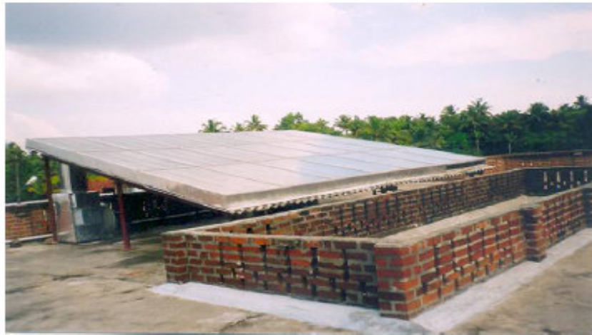
Figure 1.3. Another solar air heater used by Sreekumar who made the techno-economic analysis of it. (Source: Sreekumar, 2010)
