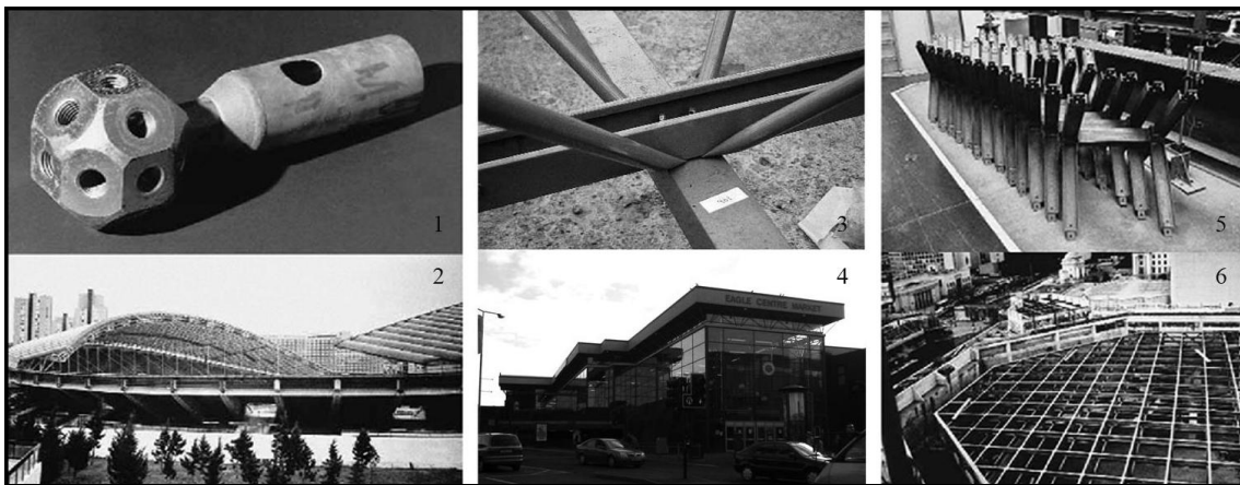
1-2. Standart Mero KK, used in stadium, Split 3-4. Harley/Conder Harley nodeless joint, used in Eagle Center Market in Derby 5-6. CUBIC Space Frame modules applied in Int. Convention Center, Birmingham
