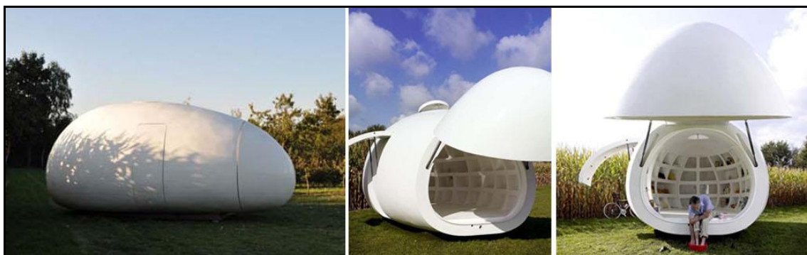
Figure 1.7. Small capsule building for office usage (Source: Arnewde, 2011)
