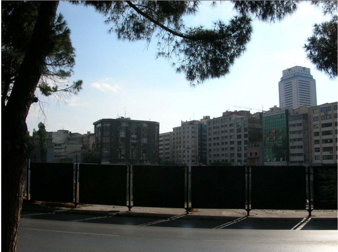
Figure 4.24. Abandoned Construction Site
