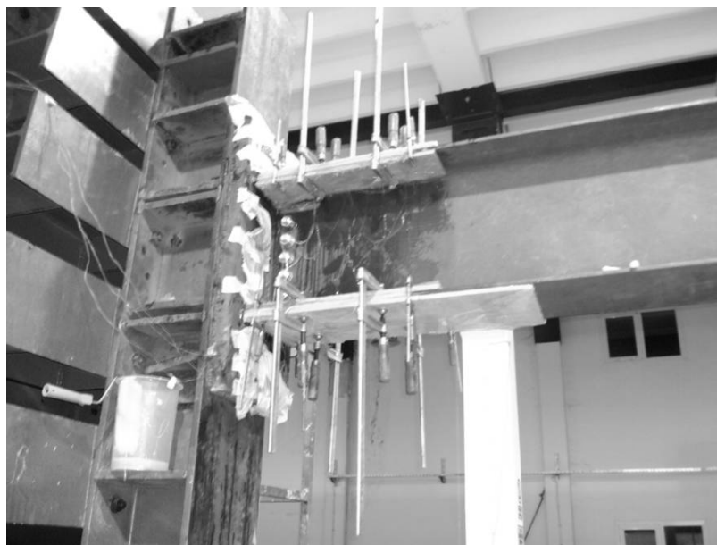
Figure 3.15. Clapping GFRP with Wood Plates
