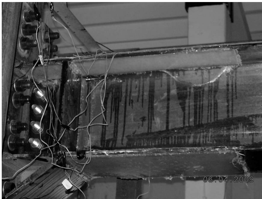
Figure 3.19. HE400AA GFRP2 Beam
