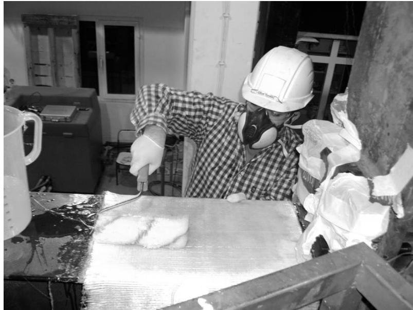
Figure 3.14. Direct Wet Lay-up Application
