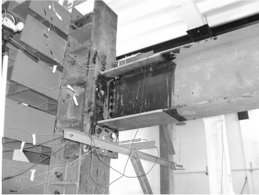
Figure 3.23. HE500AA GFRP1 Beam
