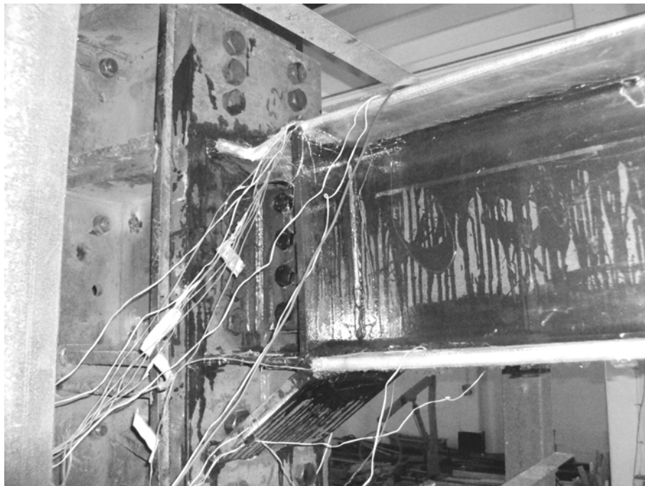
Figure 4.18. HE400AA GFRP3 Beam Top Flange at 0.043 rad of Rotation
