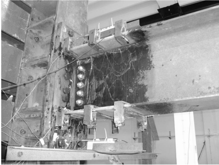
Figure 3.25. HE500AA GFRP2 Beam
