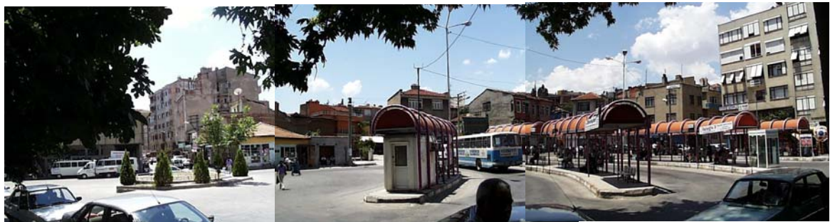
Figure 5.55 A view from Zağnos Paşa Mosque towards the square on its west, the problem of enclosure, and the impairment of spatial unity with bus stops.
