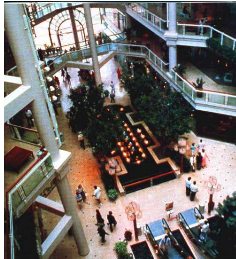
Figure 2.18 The Gallery at Harborplace, Baltimore, Maryland, interior. (Source: Altoon, R. A., International Shopping Center Architecture, International Council of Shopping Centers, 1996. p.117)
