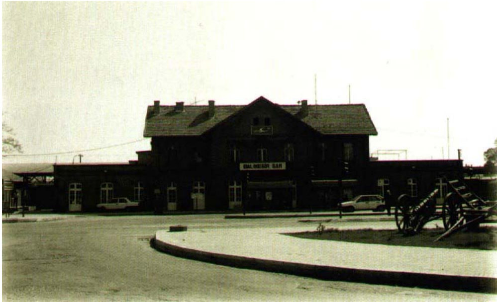
Figure 5.2 Station Building in Balıkesir. (Source: Yerce Photography, Balıkesir.)
