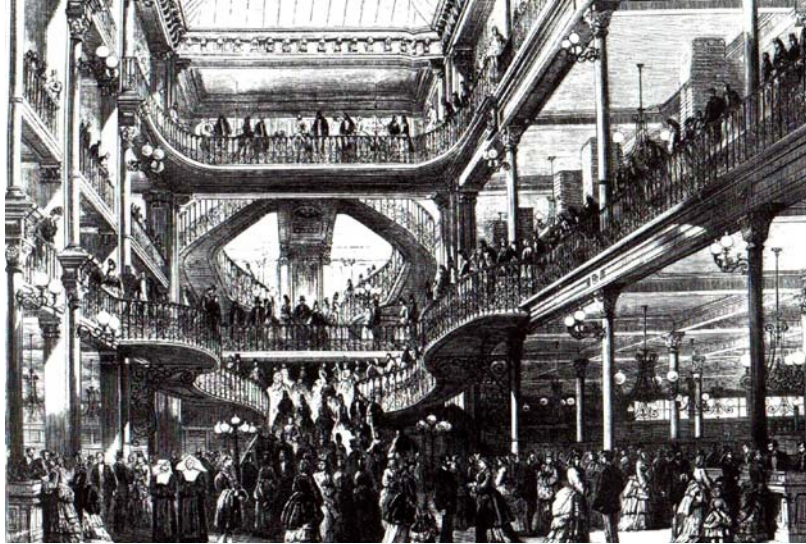
Figure 3.22 Paris, Bon Marche, staircase and glass roof.
