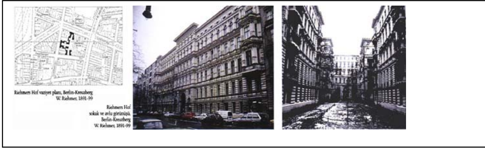
Fig. 2. Adjacent Apartment Houses, Architect W. Riehmer, Riehmers Hof, Berlin, 1891-99
