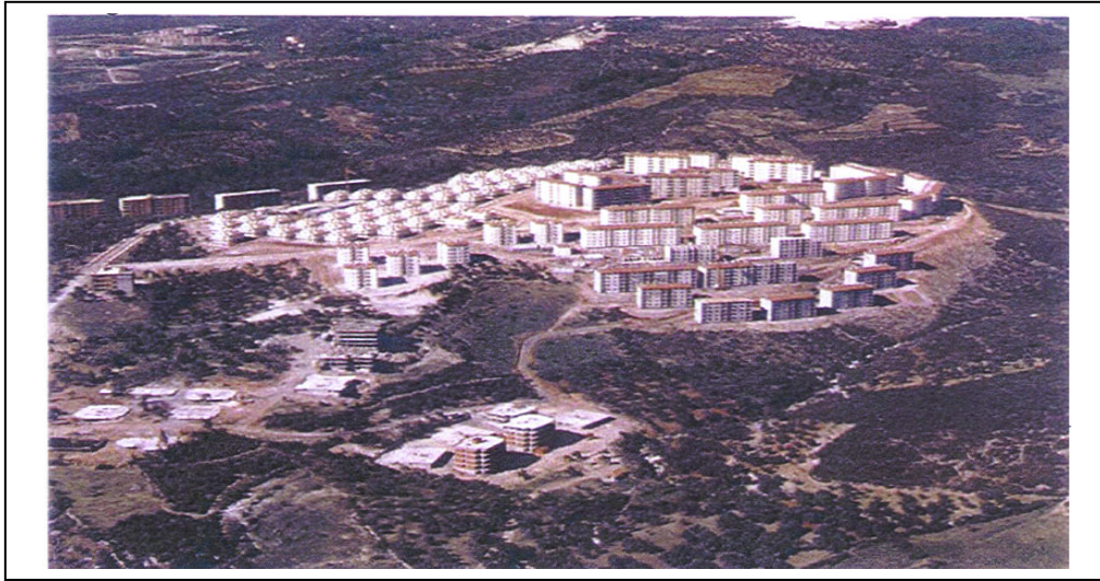
Fig. 32. Modern Satellite Settlements-Mass Housing Projects,
