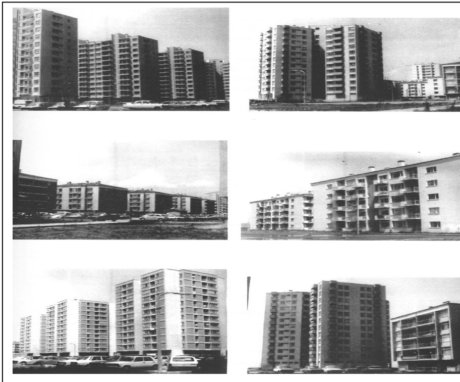
Fig. 55. Mass Housing Projects, Emlak Bank, Bostanlı- Izmir, 1981
