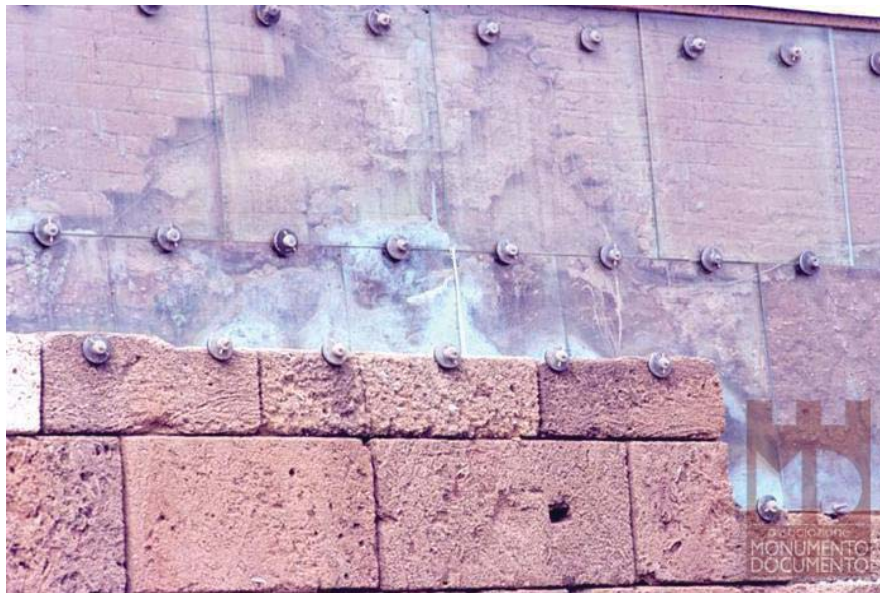
Figure 3. 20. Transparent sheets that were mounted on the façade to prevent rain, caused an ideal microclimate for plants and animals. (Source: http://www.unipa.it/monumentodocumento/villadelcasale/lastre_vetro.html )
