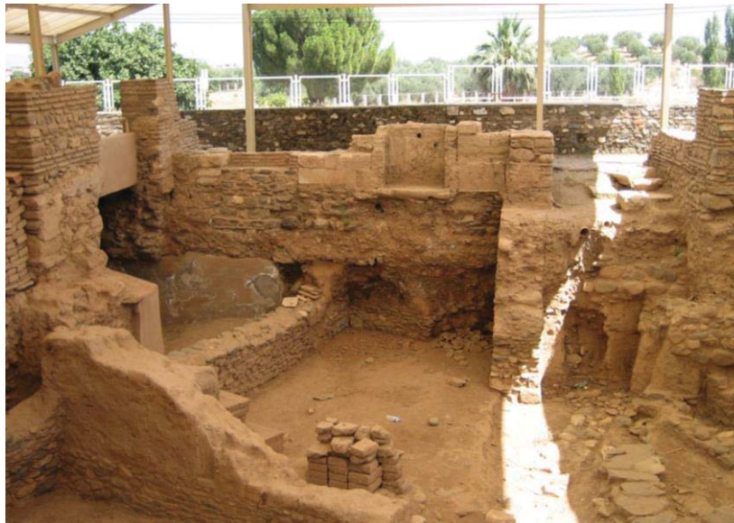
Figure 3. 4. Rising damp due to faulty gutter system.
