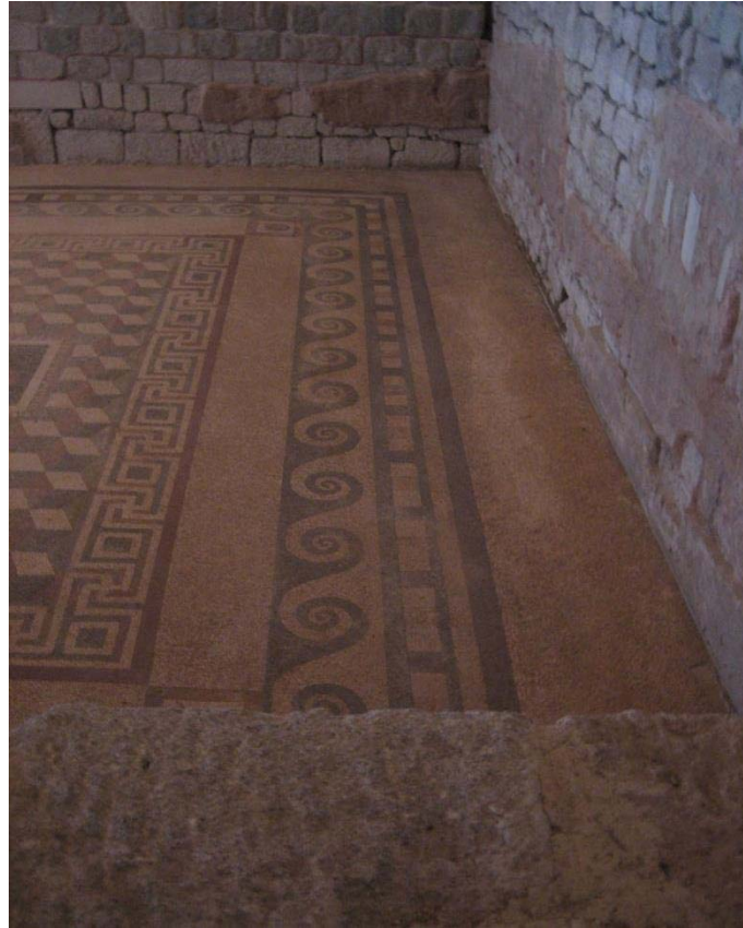
Figure 3. 3. Color alterations due to drainage problems.
