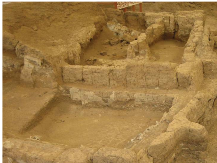
Figure 3. 9. Collapse of mudbrick walls due instable microclimate at south shelter.
