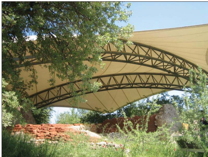
Figure 2. 1. Protective shelter in Troy, Turkey.
