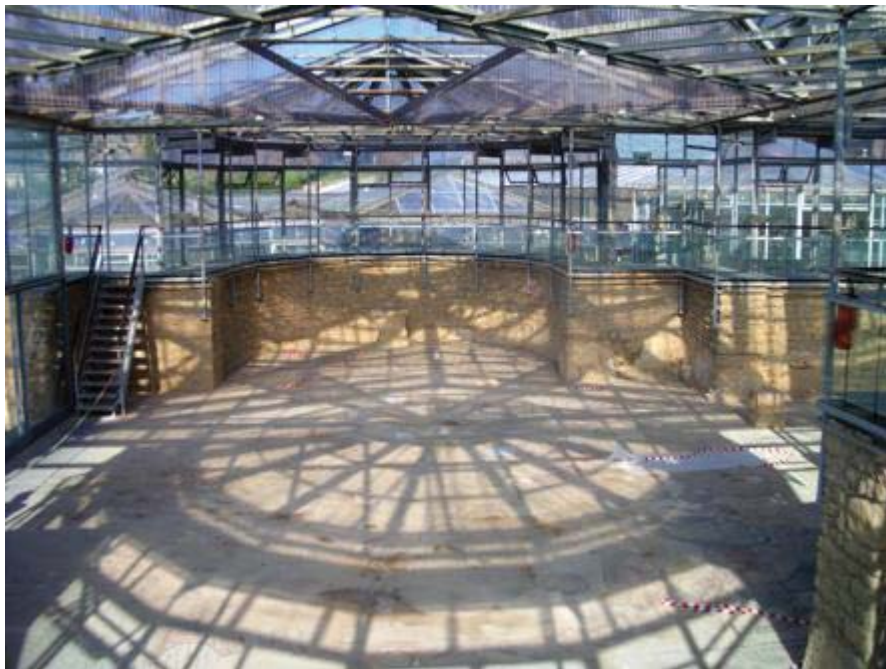
Figure 3. 19. The shading elements fail to prevent direct solar gain and heat built up in the Roman Villa at Piazza Armerina (Sicily, Italy). (Source: http://www.studiogionatarizzi.com/progetto/galleria/30/#18 )
