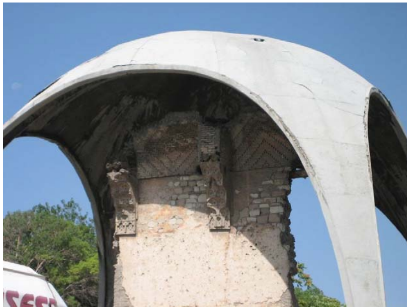
Figure 3. 13. Salt crystallization on the glazed bricks.
