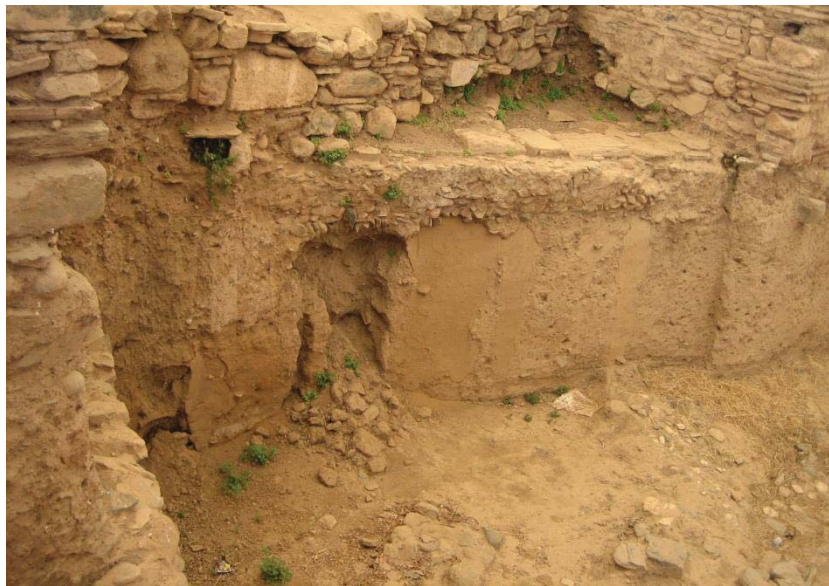
Figure 4. 2. Plant growth on the mudbrick fortification wall at the Archaic and late Roman remains at Sardis (Turkey).
