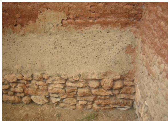
Figure 3. 15. Holes by wasps and arthropods at the Citadel Wall and the Megaron at Troy (Turkey).
