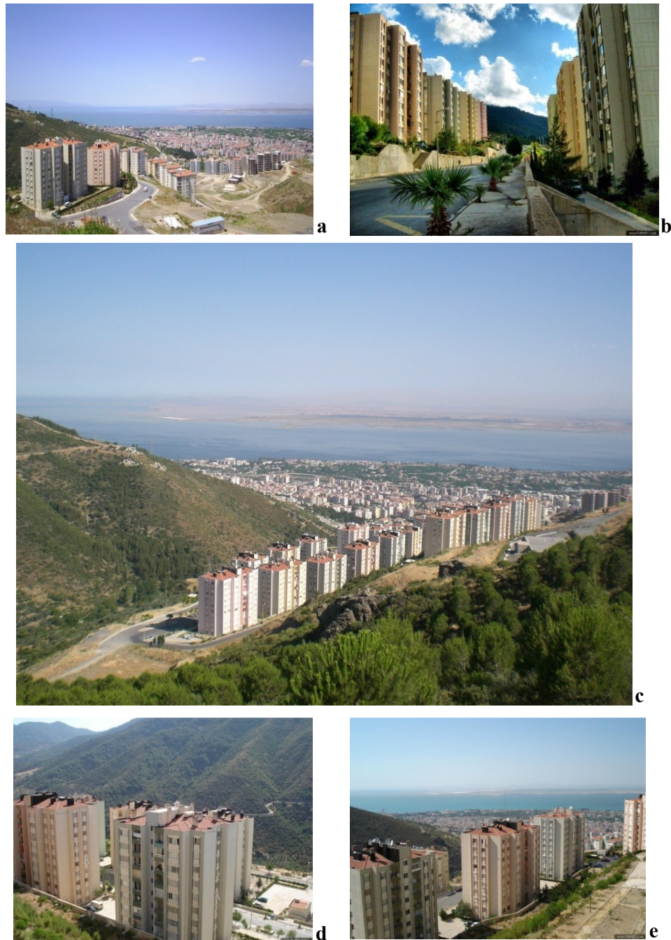
Figure 5.23. Narbel Mass-Housing, Narlıdere, Izmir, 1997-1999: a. , b. , c. , d. Views from the settlement (Sources: a. Panoramio 2009b; b. WowTurkey 2009 [photograph by Cem Tamer]; c. Panoramio 2009a [photograph by Saim Gülderen]; d. , e. WowTurkey 2006 [photographs by Orkun Kara])
