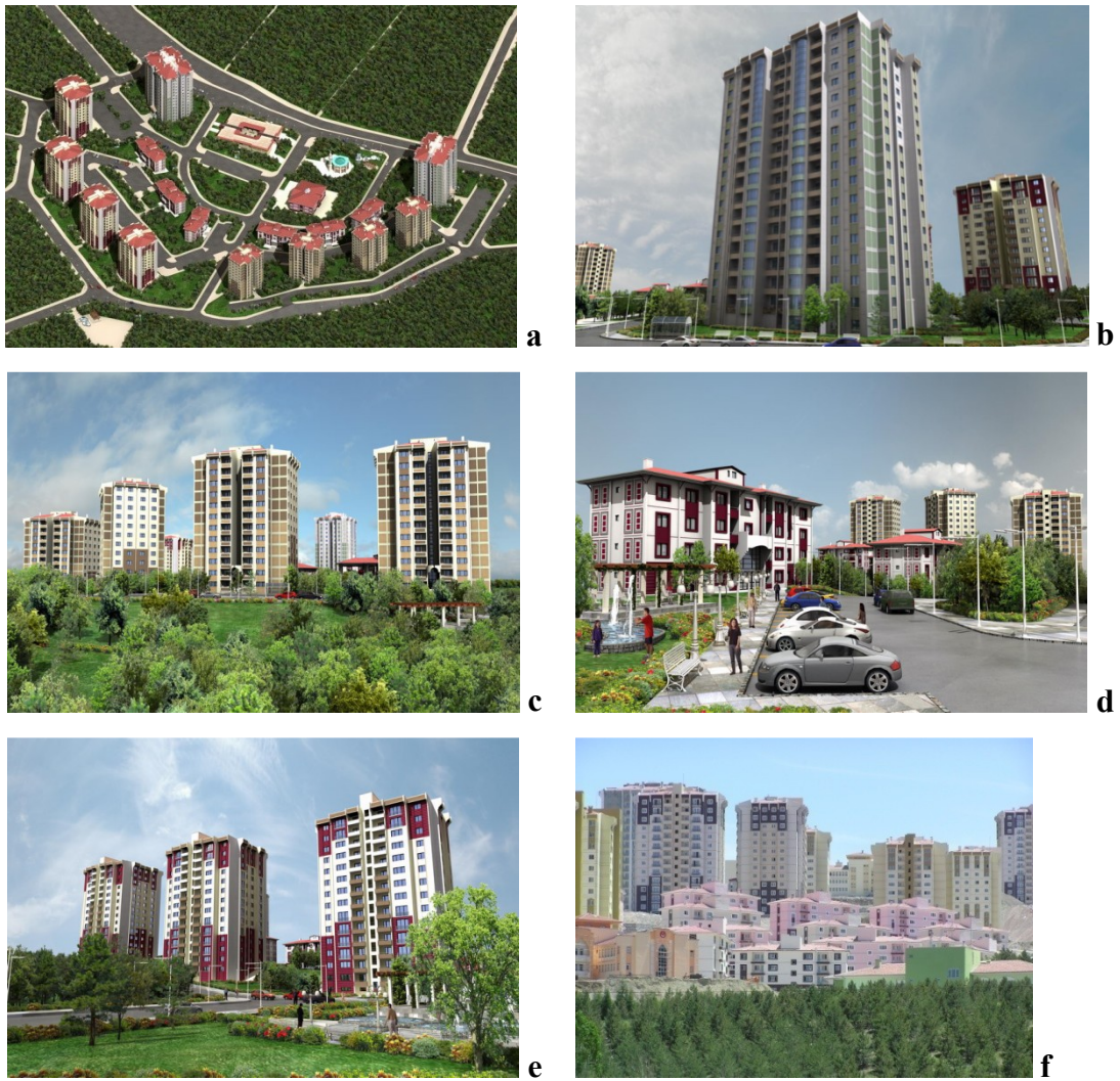
Figure 3.8. Turkuaz Vadisi Mass-Housing, Turkuaz Vadisi, Ankara, 2007-2011: a. , b. , c. , d. , e. 3D modelings; f. View from the settlement (Sources: a. , b. , c. , d. , e. İnşaat Dergisi 2011; f. Panoramio 2008)
