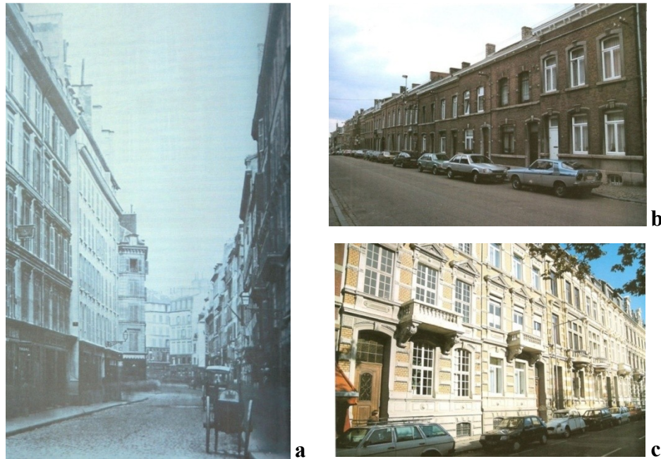
Figure 2.1. Housing typologies in Europe at the beginning of the twentieth century: a. Apartments in Paris; b. Luttichen Strasse, Aachen, Belgium; c. Frankenberger Viertel, Aachen (Sources: a. Sey 1999, 286; b., c. Sey 1999, 285)
