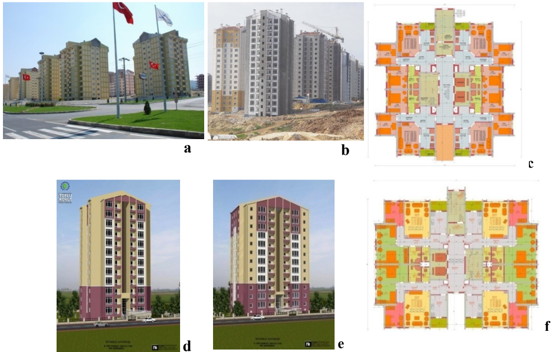
Figure 2.16. TOKI Kayabaşı project, Kayaşehir, Istanbul, 2008-2012: a. A view from the settlement; b. A view from the construction phase; c. Floor plan of B Block; d. 3D-render view from B Block; e. 3D-render view from C Block; f. Floor plan of C Block (Sources: a. İnşaat Dergisi 2009; b. Panoramio 2012 [photo by Seyid Can, 2010]; c., d., e., f. TOKI 2011a)
