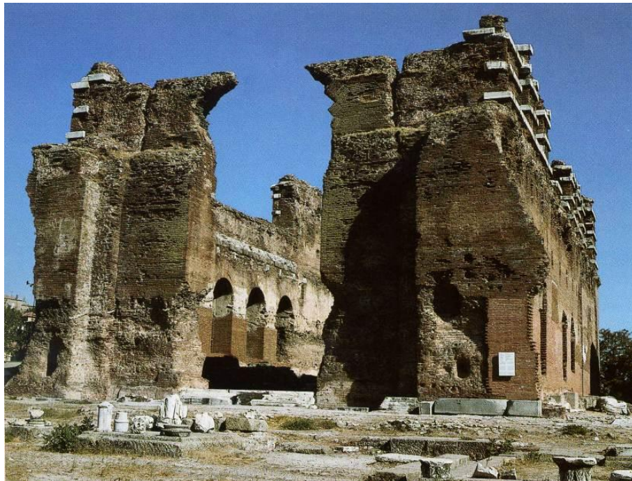
Figure 1.21. Kızıl Avlu at Pergamon constructed by mortared brick throughout (Source: Radt 2002, p.198)
