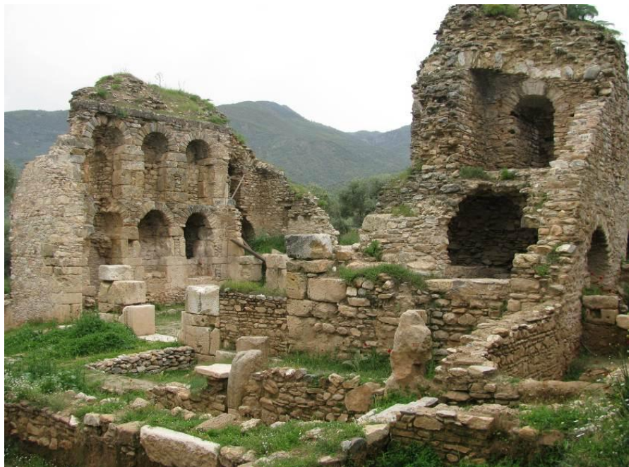
Figure 1.20. The library at Nysa constructed of mortared rubble throughout
