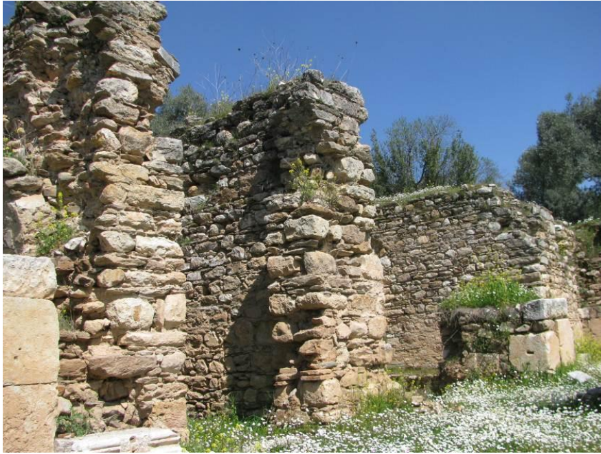
Figure 1.19. The walls of agora at Nysa comprised of mortared rubble throughout
