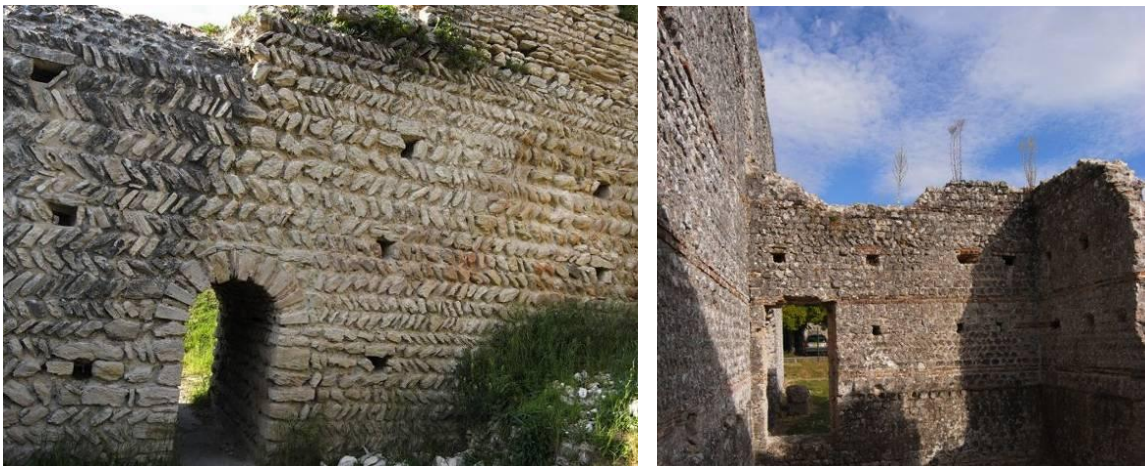
Figure 1.12. Opus spicatum in the Mansio in Thésée (Source: Montjoye 2012)
