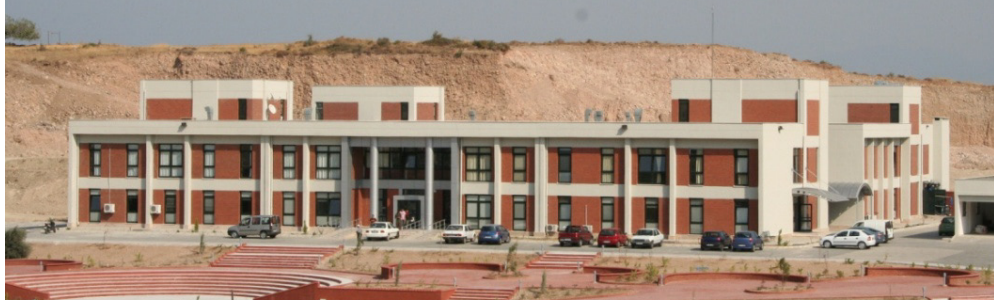
Figure 16. View of MEDICO Building (west & south facades)
