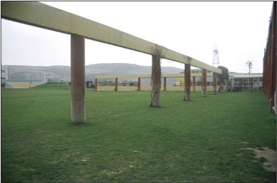
Figure 37. In the garden of Işıkkent ES, a row of columns provides a buffer zone in front of the windows of classrooms.
