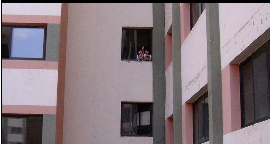
Figure 56. The emergency stairs of Building A of Fatih ES.
