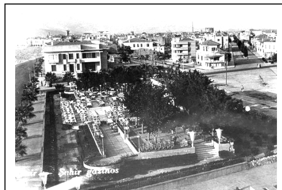
Figure 4.23. The tee garden before the construction of City Hotel; (source: IKEMA)
