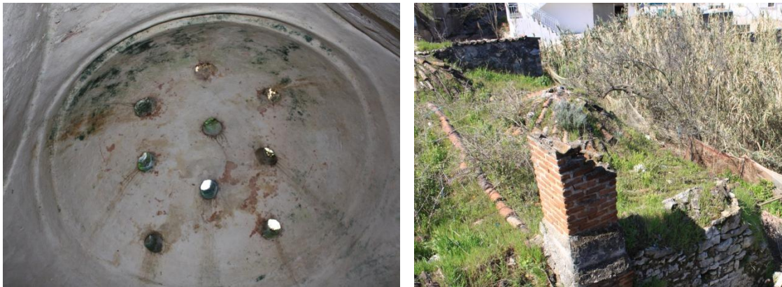
Figure A.102. Özbek Köyü Hamamı, interior and exterior views of northwest halvet dome.
