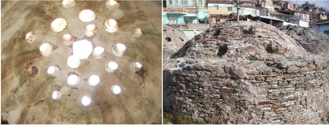
Figure A.16. Tire Hekim Hamami, interior and exterior views of halvet dome of the women's section.
