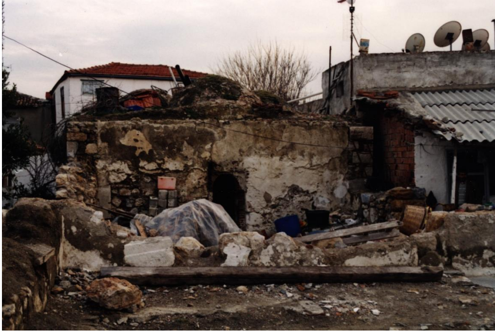
Figure A.75. Sığacık Kaleiçi Hamam, a general view of superstructure (2004).
