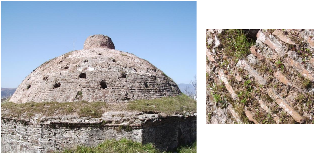
Figure 3.27. In Tire Yalınayak Hamamı men's section sıcaklık main space dome using the bond type of “horizontal stacking of long faces on the bottom for a few rows and short faces on top in parallel rows”.
