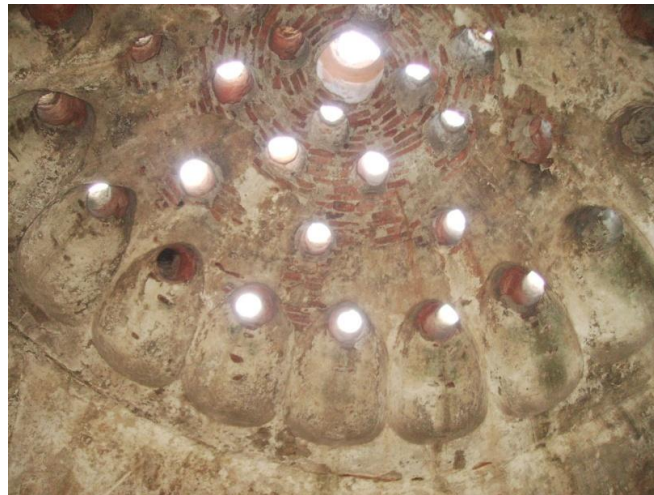
Figure 2.13. Segmented profiles in the horizontal direction located in the halvet dome of Tire Hekim Hamamı men's section.
