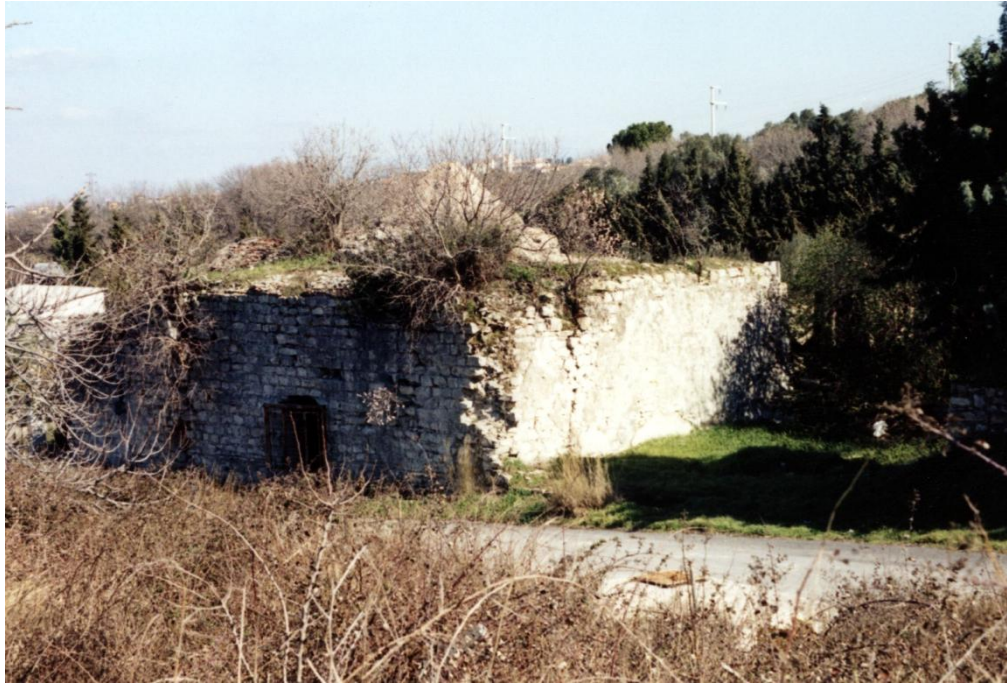
Figure A.89. Urla Kamanlı Hamamı, a general view of superstructure (2004).
