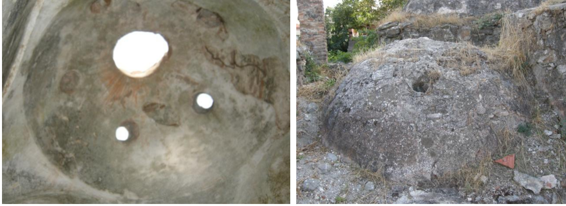
Figure A.73. Seferihisar Küçük Hamam, interior and exterior views of northeast halvet dome.
