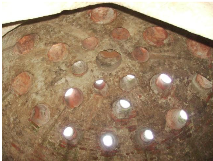
Figure 3.50. In Tire Hekim Hamamı men's section southeast halvet dome, for the purpose of space lighting penetrations the use of terracotta pipes in the brick bond.
