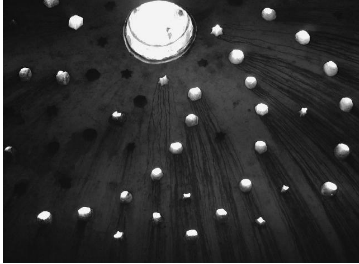
Figure 3.49. The use of hexagonal oculi in spiral geometrical order with star shaped in between randomly in the sıcaklık main space dome of Tire Yalınayak Hamamı men's section.
