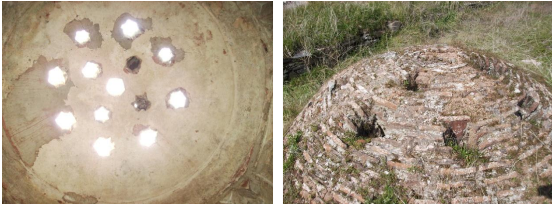
Figure A.43. Tire Yalınayak Hamamı men's section, interior and exterior views of the west corner halvet dome.
