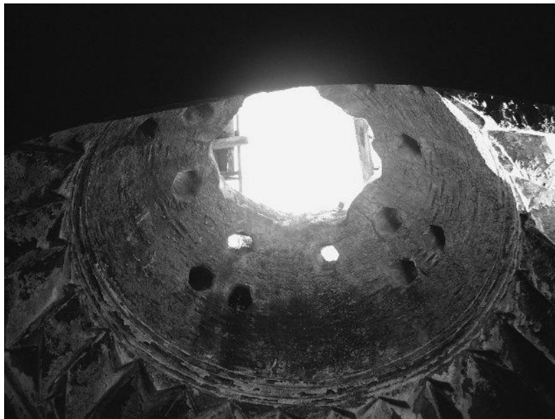
Figure 3.48. The use of hexagonal oculi in ternary and single orders alternately in the sıcaklık main space dome of Tire Tahtakale Hamamı.
