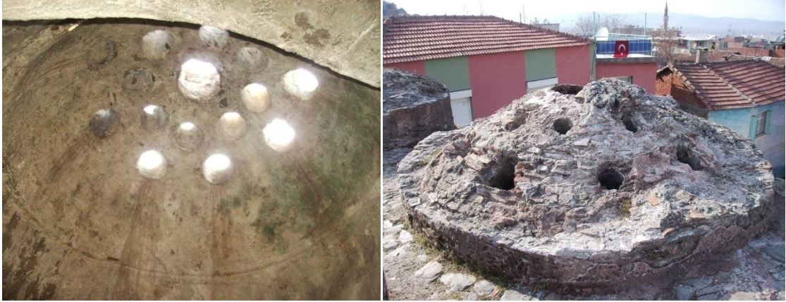
Figure A.14. Tire Hekim Hamamı, interior and exterior views of ılıklık / sıcaklık main space dome of the women's section.
