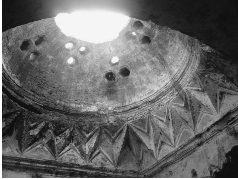
Figure 3.47. The use of hexagonal oculi in ternary type in the ılıklik main unit dome of Tire Tahtakale Hamamı.
