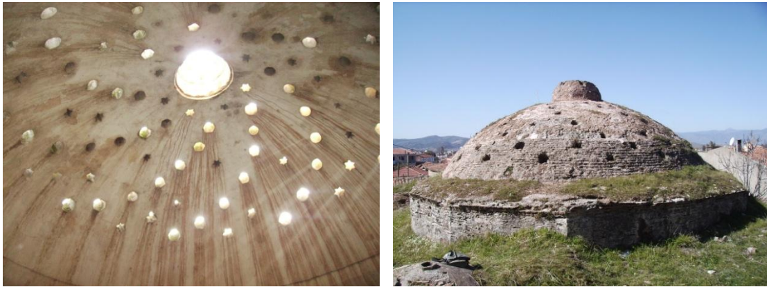
Figure A.42. Tire Yalınayak Hamamı men's section, interior and exterior views of sıcaklık main space dome.
