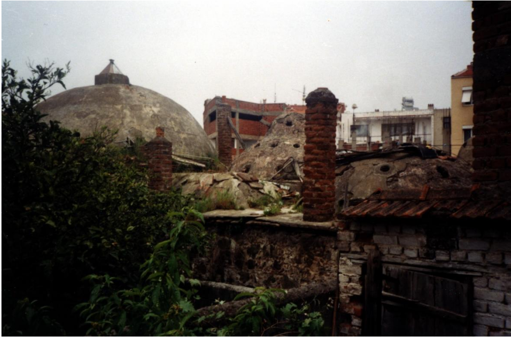
Figure A.62. Seferihisar Büyük Hamam, a general view of superstructure (2004).
