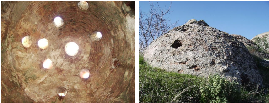
Figure A.61. Düzce (Hereke) Hamamı, interior and exterior views of southeast halvet dome.
