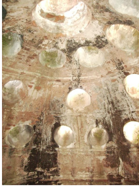
Figure 2.16. Truncated-octagonal pyramidal, on the top circular depressed profiles in the dome of Urla Hersekzade Ahmet Paşa Hamamı women's section sıcaklık main space.
