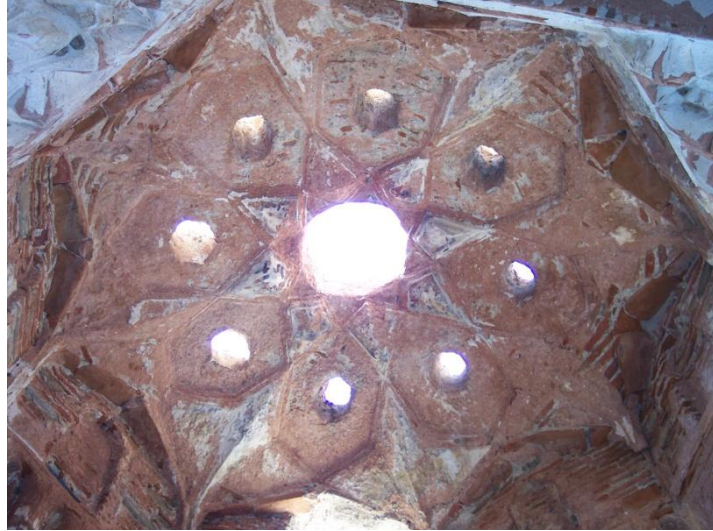
Figure 3.50. In Tahtakale Hamamı, in the interior surface of the depressed pyramidal dome of northwest iwan of sıcaklık main space, the use of eight-strand star ornament created with horasan plaster and placed oculus in each strand.
