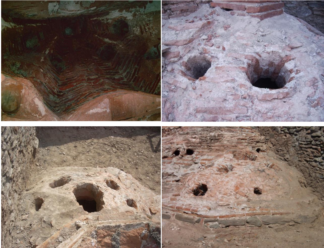
Figure A.8. Tire Tahtakale Hamami, interior and exterior views of rectangular planned segmented iwans' semi-domes.
