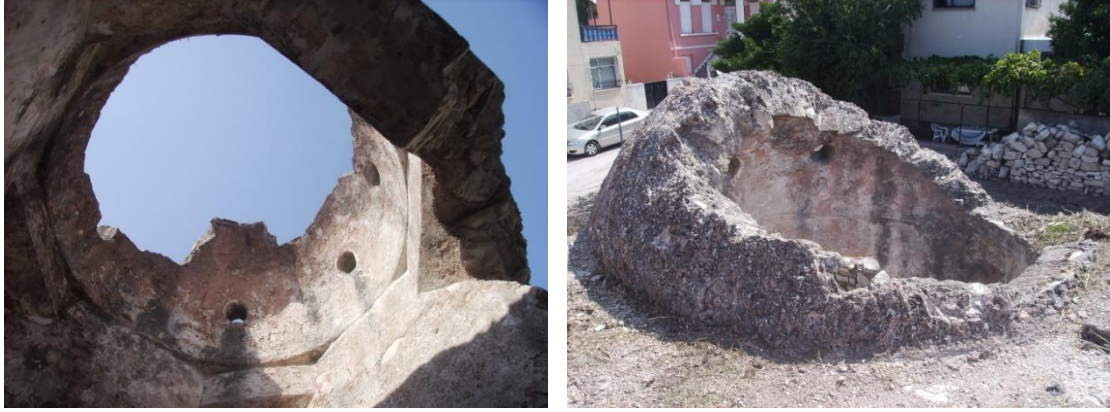
Figure A.82. Urla Hersekzade Ahmet Paşa Hamamı, interior and exterior views of ılıklık dome in the men's section.
