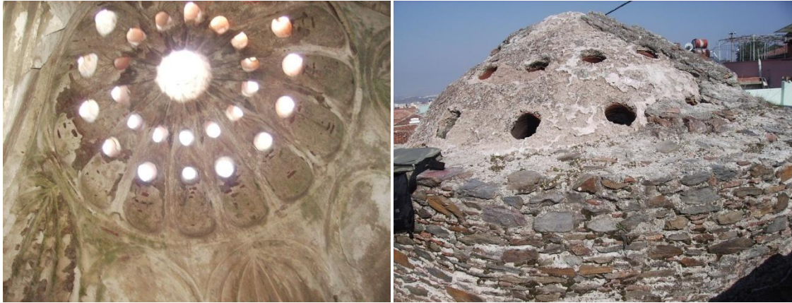
Figure A.17. Tire Hekim Hamamı, interior and exterior views of ılıklık / sıcaklık main space dome of the men's section.
