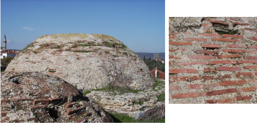
Figure 3.25. In Düzce (Hereke) Hamamı soyunmalık dome using the bond type of “horizontal and adjacent stacking of the short side faces in parallel rows”.
