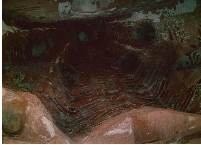
Figure 2.15. Segmented semi-circular profiles in the semi-dome of east side iwan unit of Tire Tahtakale Hamamı sıcaklık main space.
