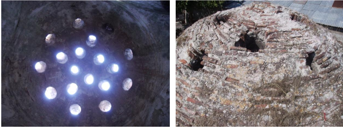
Figure A.88. Urla Hersekzade Ahmet Paşa Hamamı, interior and exterior views of southwest halvet dome in the women's section.
