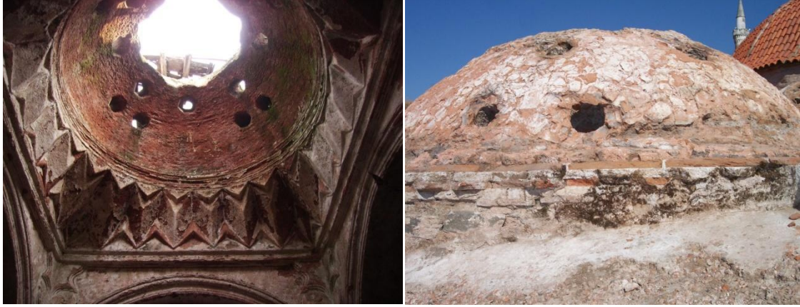
Figure A.7. Tire Tahtakale Hamamı, interior and exterior views of sıcaklık main space dome.
