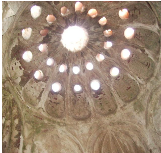
Figure 2.14. Segmented profiles in the vertical direction located in the ılıklik dome of Tire Hekim Hamamı men's section.
