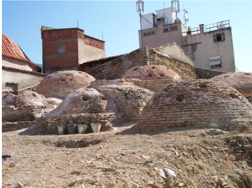
Figure A.1. Tire Tahtakale Hamamı, the general view of superstructure (2008).
