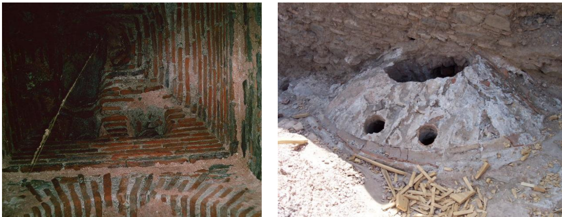
Figure A.4. Tire Tahtakale Hamami, interior and exterior views of aralık dome.
