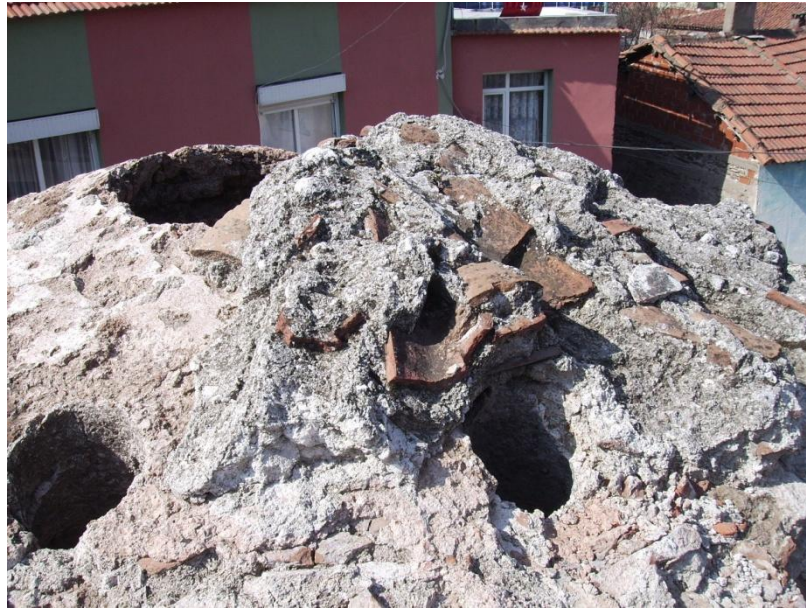
Figure 3.65. In the dome of ılıkılık/sıcaklık main space west sub-unit of Tire Hekim Hamamı women's section, the use of horasan mortar including small and large pieces of bricks, stones, and tiles with traditional Turkish tiles covered on the exterior.
