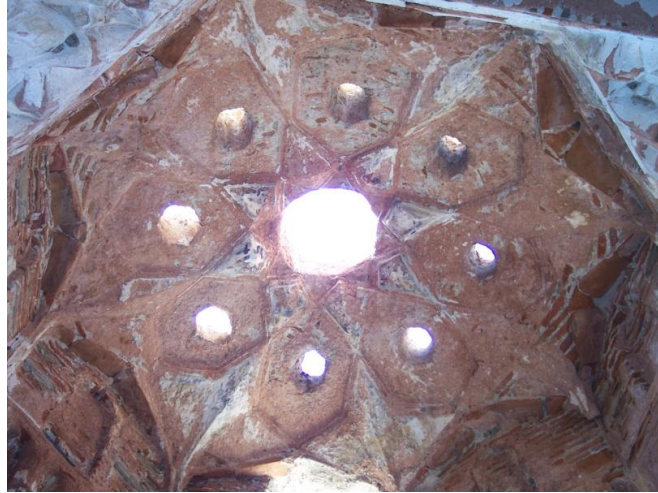
Figure 2.18. Octogonal-pyramidal profiles in the square planned dome of northwest iwan of Tire Tahtakale Hamamı men's section.
