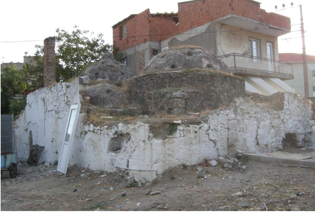
Figure A.70. Seferihisar Küçük Hamam, a general view of superstructure (2008).
