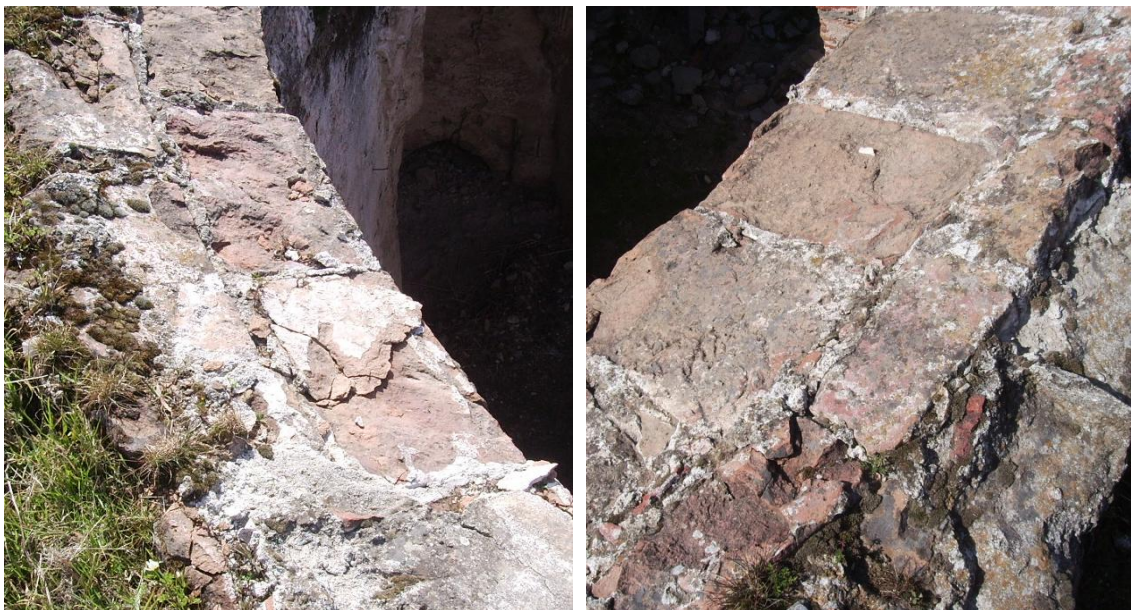
Figure 3.31. In Tire Karagazi Hamamı men’s section sıcaklık main space dome using the bond type of “in vertical sequential stacking of long/short faces on interior, horizontal stacking of the long faces on exterior surface”.
