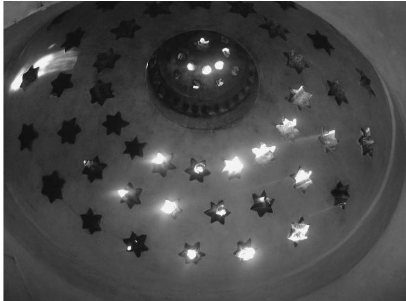
Figure 3.52. In Tire Eski-Yeni Hamamı men's section sıcaklık main space dome, the use of star shaped oculi in circular three rows and hexagonal shaped oculi in two rows on the lighting cupola at the top of dome.
