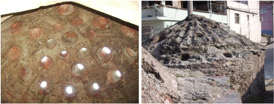
Figure A.18. Tire Hekim Hamami, interior and exterior views of southeast halvet dome of the men's section.
