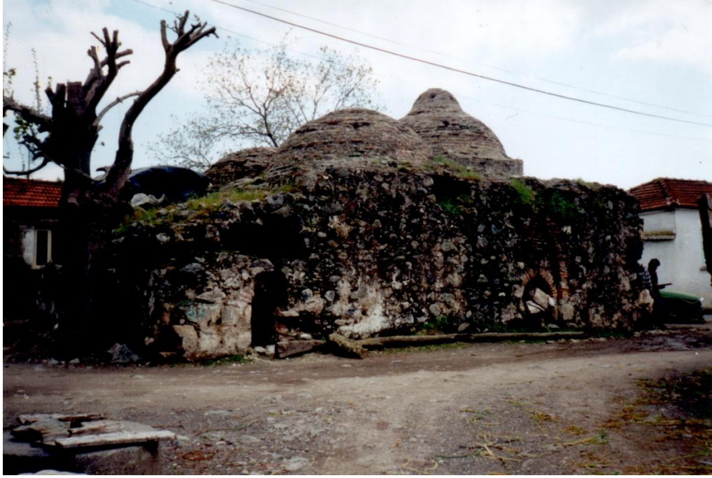
Figure A.52. Ulaş Hamamı, a general view of superstructure (2004).
