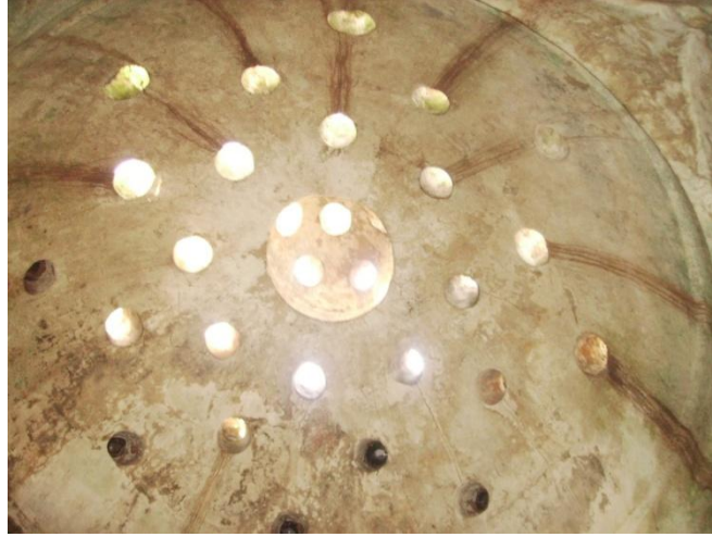
Figure A.26. Tire Mehmet Ağa Hamamı men's section, interior view of southwest halvet dome.
