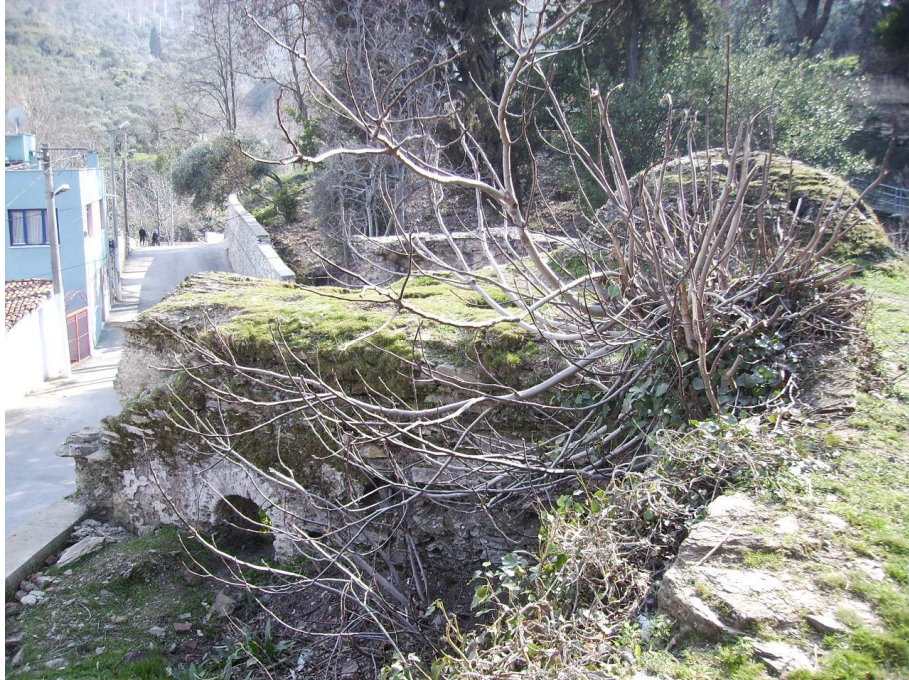
Figure A.20. Tire Şeyh Hamamı, general view of superstructure (2008).
