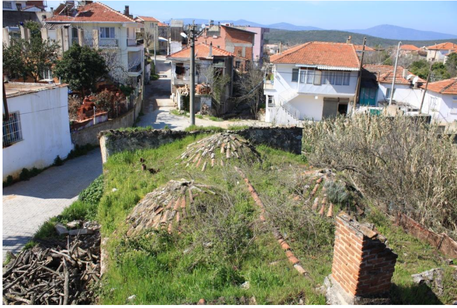
Figure A.99. Özbek Köyü Hamamı, a general view of superstructure (2008).
