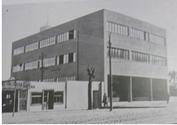
Figure 5.44. Sedad Hakkı Eldem, Electric Company (Source: Mimar June, 1934: 160)
