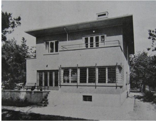
Figure 5.38. Zeki Sayar, A residence in Kalamış (Source: Arkitekt May-June, 1936: 129)
