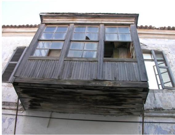
Figure 3.47. Bay window opening to sun
