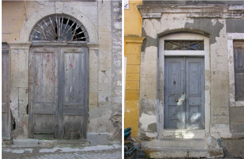
Figure 3.37 Examples of natural ventilation openings (menfez) over door detail of Alaçatı Houses
