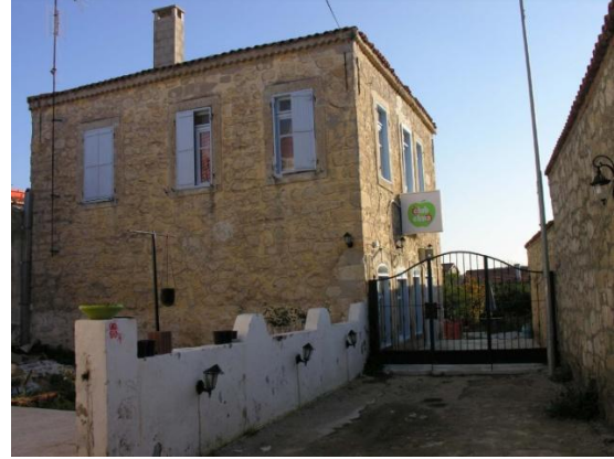
Figure 3.20. Country/ vineyard house (two stories rubble stone)
