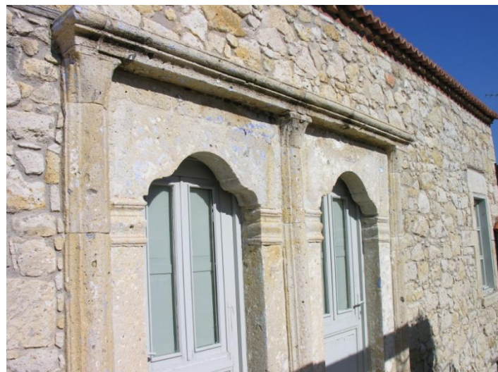
Figure 3.42. Sun control detail from outdoor terrace (hayat) door of an Alaçatı House Photo taken on 7th of Sep 2008 at 11:00
