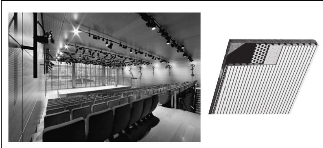
Figure 2.7 An example Helmholtz absorber and an application on the walls and ceiling in the auditorium of The Times Center [2].
