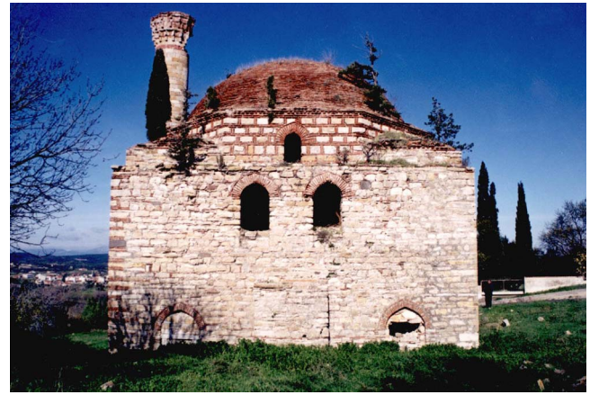
Fig. 2. South elevation view of the structure
