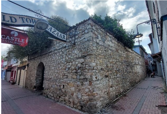
Condition Class 1: Housing (CUH13)
