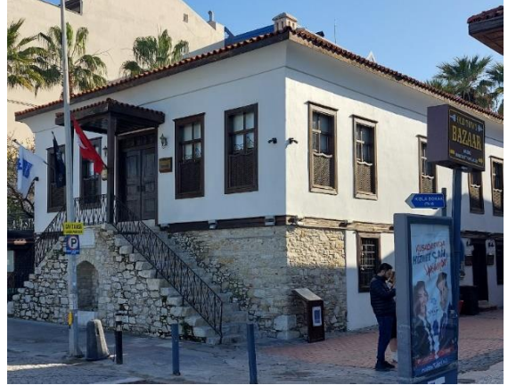
Masonry + Steel Frame: Historic School (CRP1)
