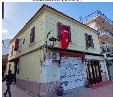
Housing Building (CRH16)
