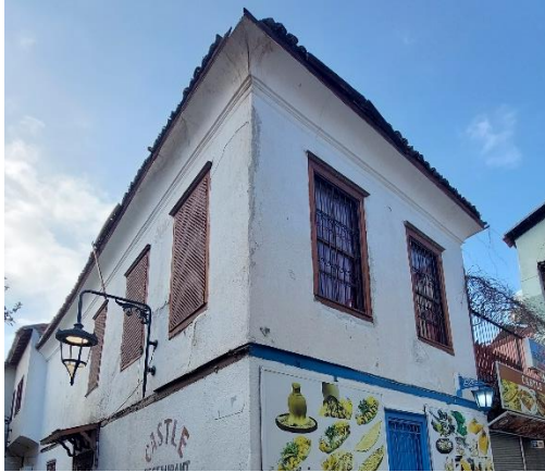
Condition Class 1: Housing (CUH14)
