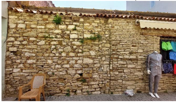
Condition Class 1: Housing (CUH2)
