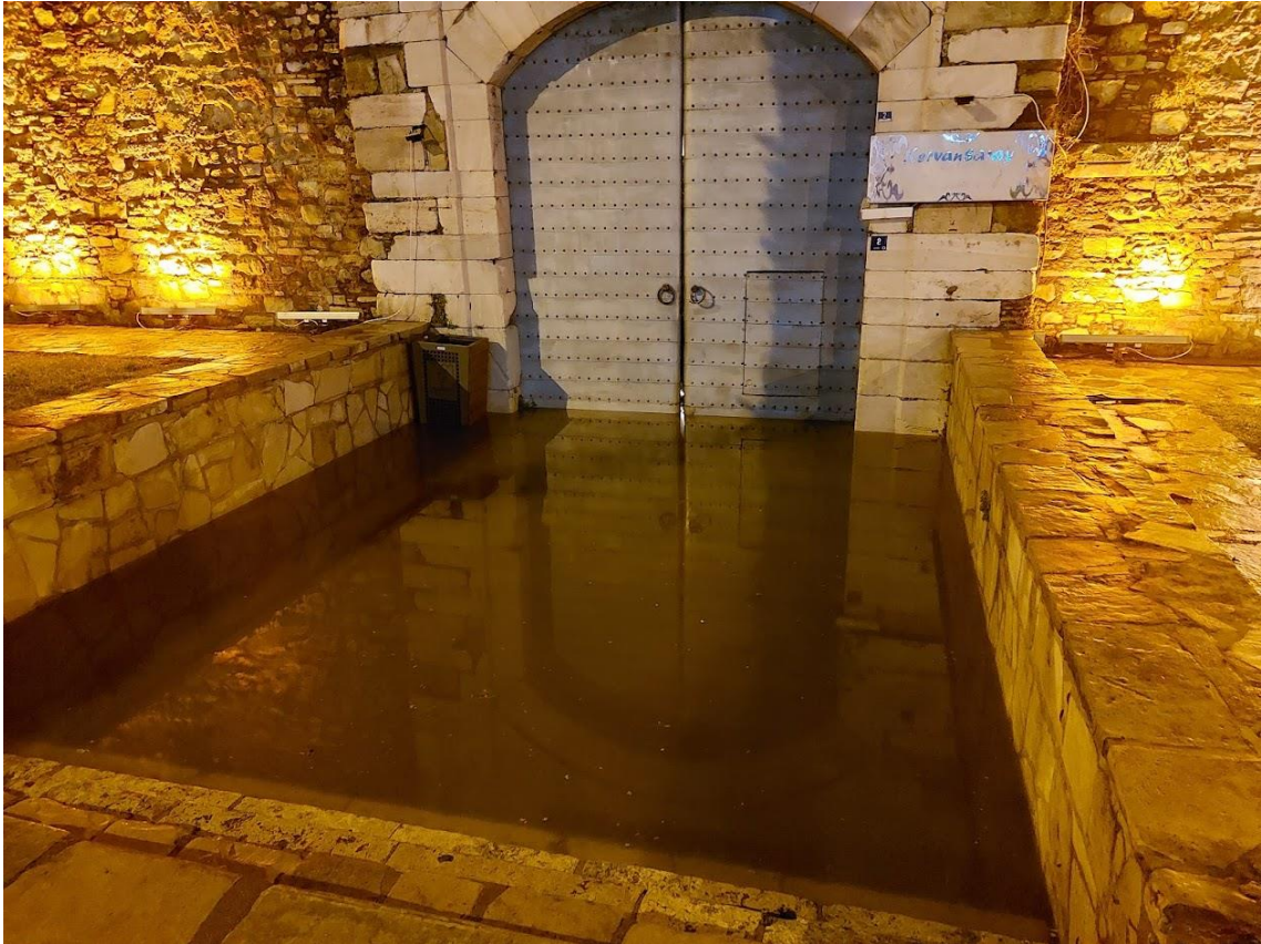
Figure 43: After Extreme Rainfall in April 2023 (Source: S. Burçak Çıkıkçı Archive, 2023)
