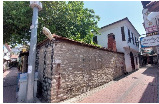
Condition Class 0: Housing (CRH9)
