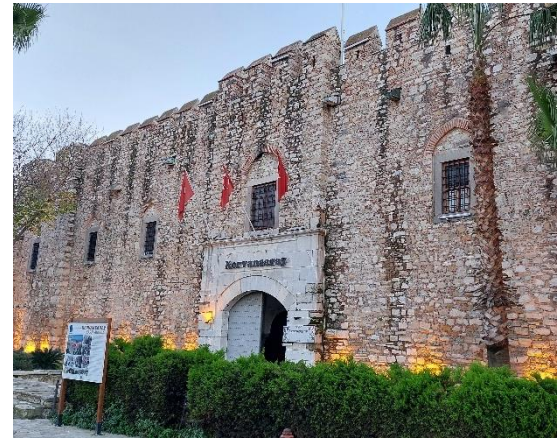
Commercial Building: Caravanserai (DRP1)
