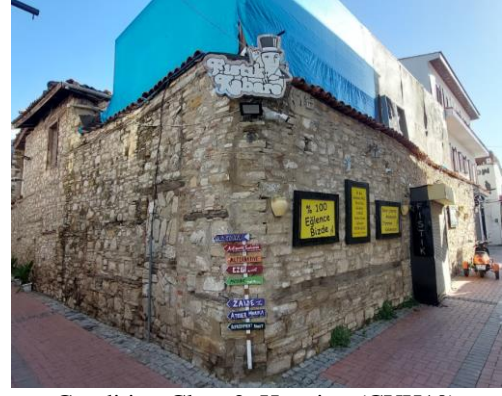
Condition Class 2: Housing (CUH10)
