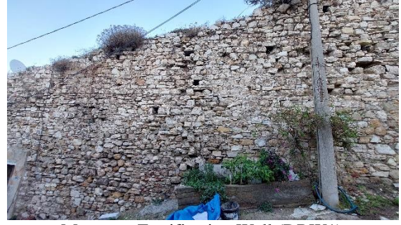
Masonry: Fortification Wall (DRW1)
