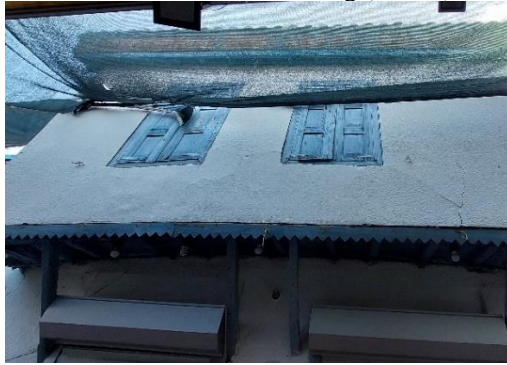
Condition Class 1: Housing (CUH14)
