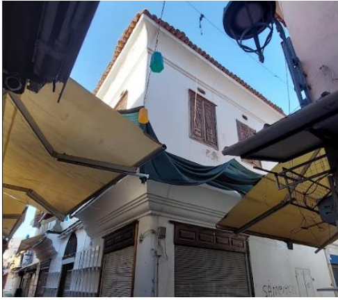
Reinforced Concrete: Housing (CRH10)
