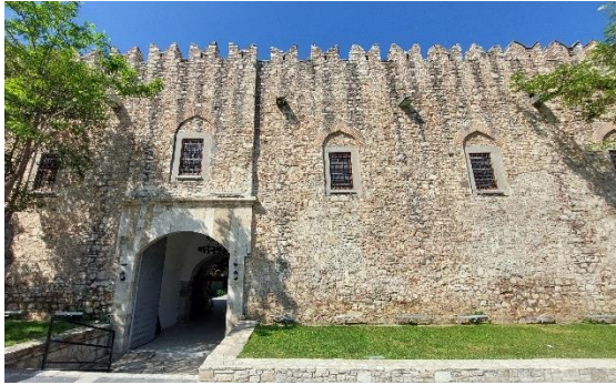
Condition Class 3: Caravanserai (DRP1)
