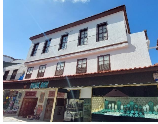
Condition Class 0: Housing (DRH1)
