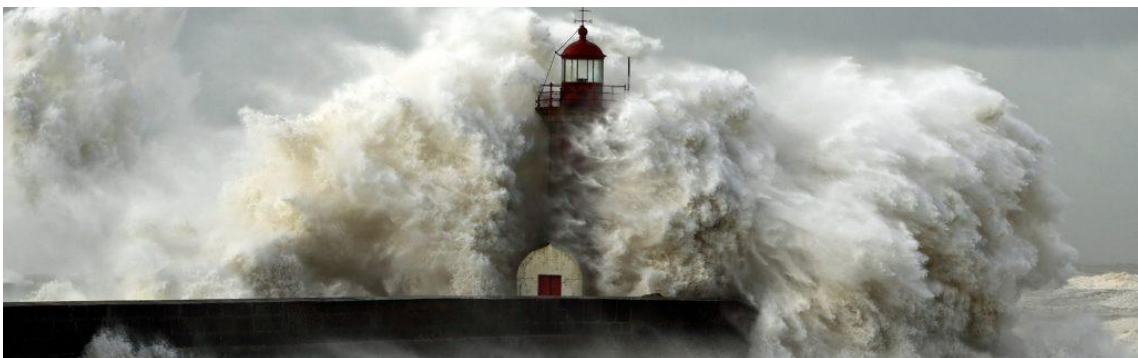
Figure 8: A storm surge affected cultural heritage. (Source: BeSafeNet, 2023)
